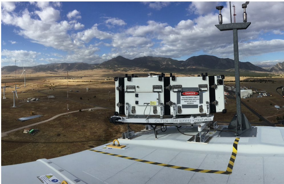
Figure 3.2: The SWE scanning lidar being installed on a rotating frame on the DOE 1.5 turbine. Photo by Andrew Scholbrock, NREL
