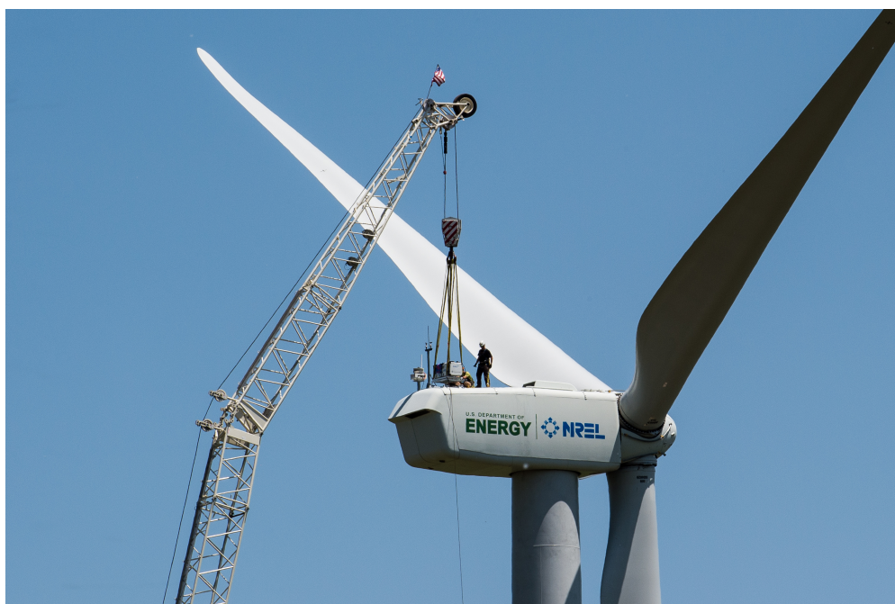
Figure 3.1: The DOE 1.5 MW turbine at the NWTC is shown with the Stuttgart Wind Energy (SWE) scanning lidar being installed. Photo by Dennis Schroeder, NREL 38271
