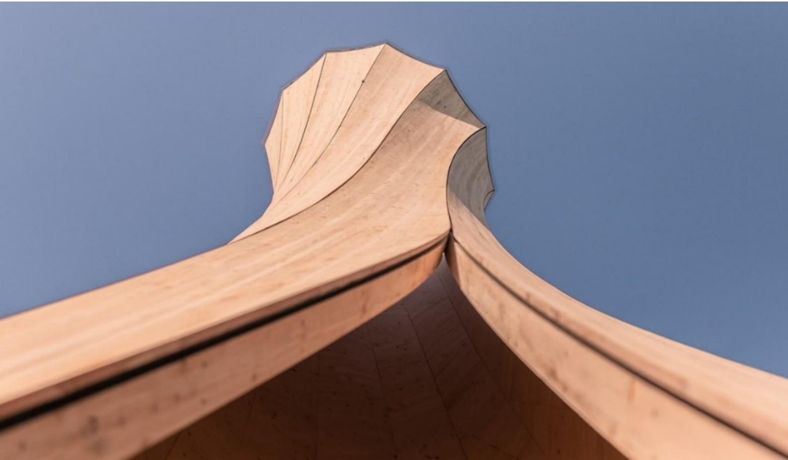
Figure 7.4: The sharp defining lines of the exterior of the Urbach Tower.
