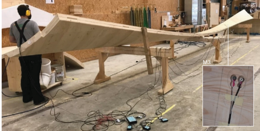
Figure 6.10: Installation of WMC sensors in the self-shaped curved components during prefabrication.
