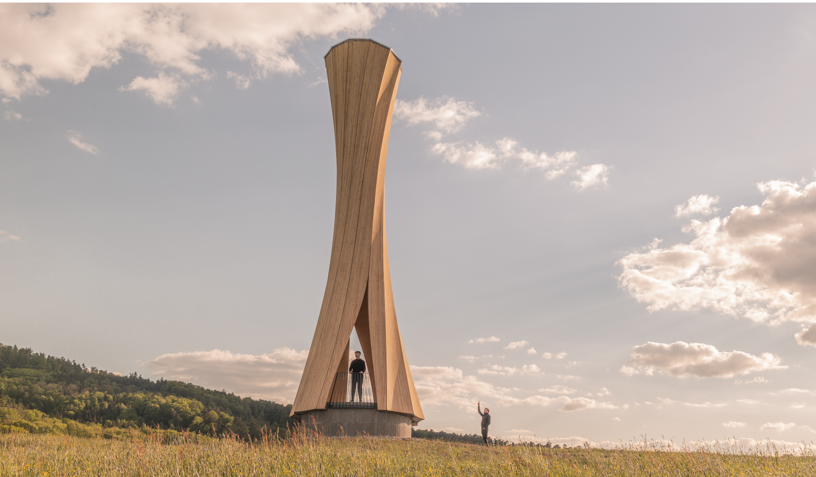
Figure 7.6: Completed structure of the Urbach Tower.
