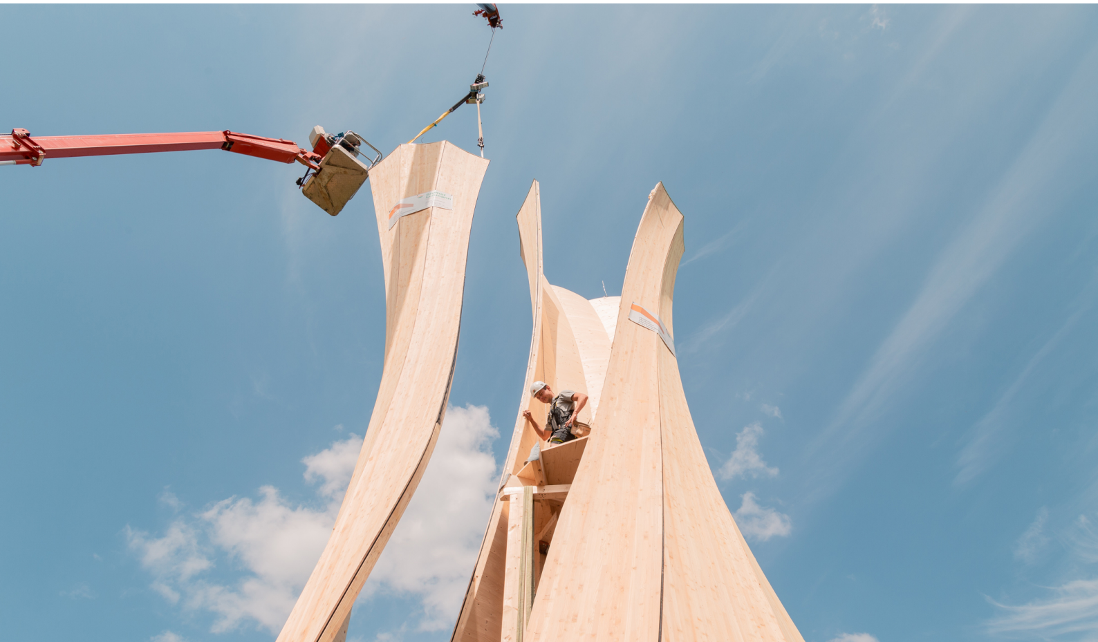
Figure 7.3: Assembly of the prefabricated curved building components on the building site.
