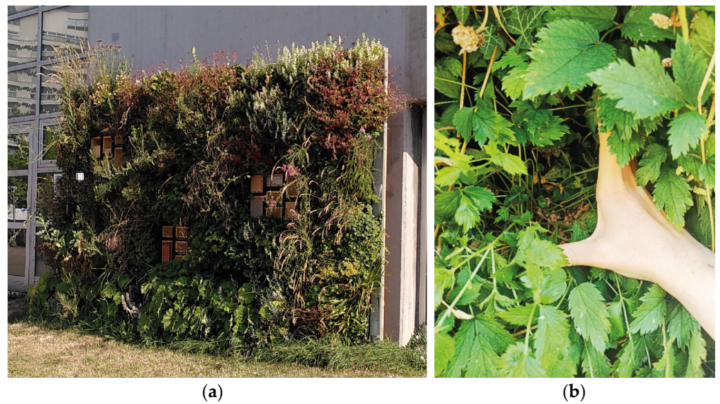
Figure 10. (a) Photograph of the plant depth in July. In response to the site conditions and the microclimate, two vertical plant layers have formed. The first layer (starting from the substrate) is formed by herbs up to a depth of 45 cm. The second layer contains plants that grow in half-light to full-light conditions, such as Cirsium arvense (field thistle), Trifolium pratense (meadow clover), and Epilobium (willowherb). (b) Detailed photograph of the planting layer in June. In the background grows Hedera helix (common ivy) and in the foreground Geranium x cantabrigiense (cranesbill).
