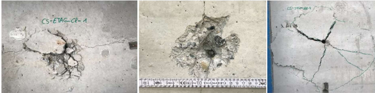
Figure 5.15. Typical failure modes of concrete screws in uncracked and cracked concrete.
