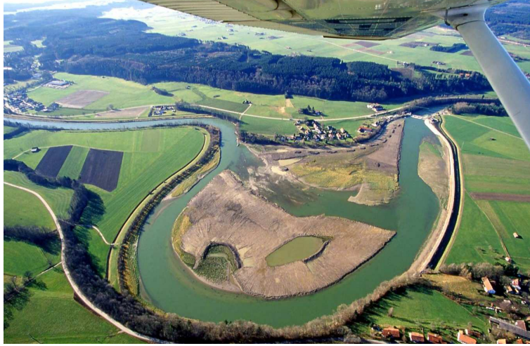
Figure 4.2: Aerial view of the Lautrach reservoir
