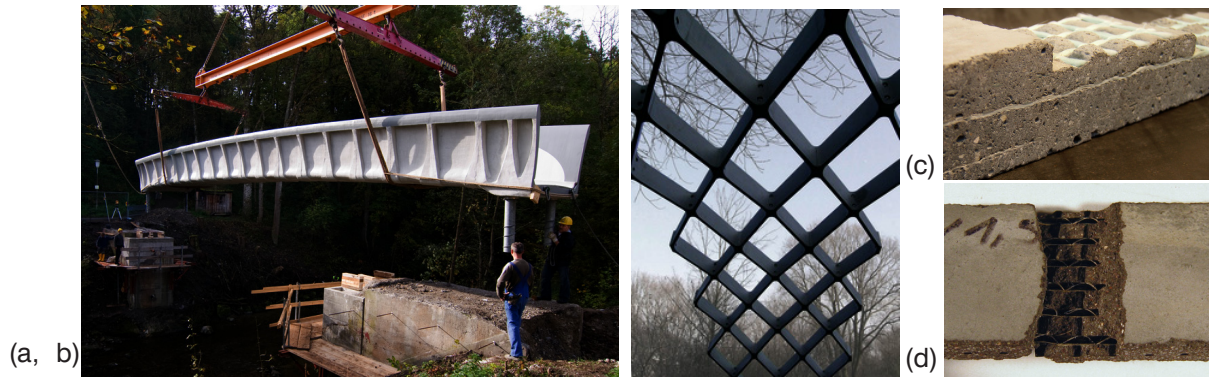
Figure 3.1: FRC structures: (a) FRC pedestrian bridge with 16m span in Kempten, Germany ( Curbach & Jesse [50] ), (b) FRC grid arch (RWTH Aachen), (c) FRC plate with a few textile layers (INNtexas Innovation Netzwerk textil e.V.), (d) FRC plate with single layer ( Hund [85] )
