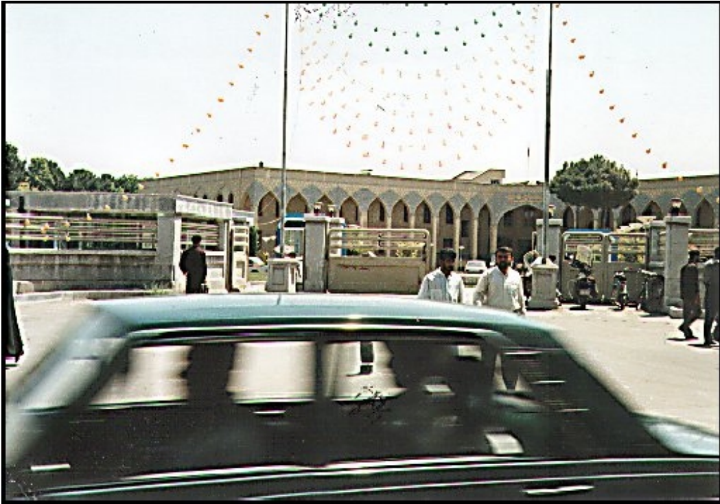
Figure 167: Construction of new buildings in traditional form. The new Administrative building in Isfahan city.
