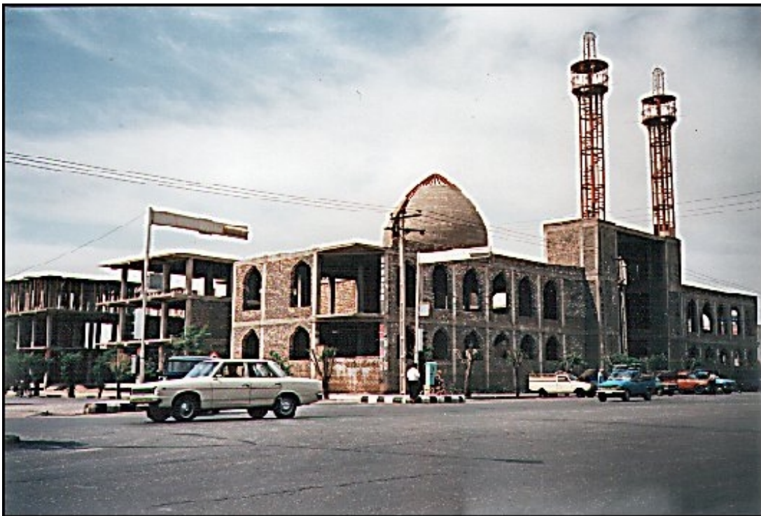
Figure 106: Exposure of traditional building characteristics of the area. Source: Author
