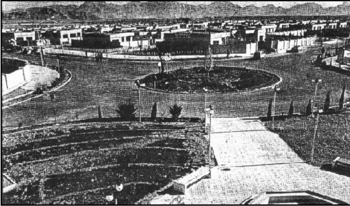
Figure 118: Majlesy new town in general view.
