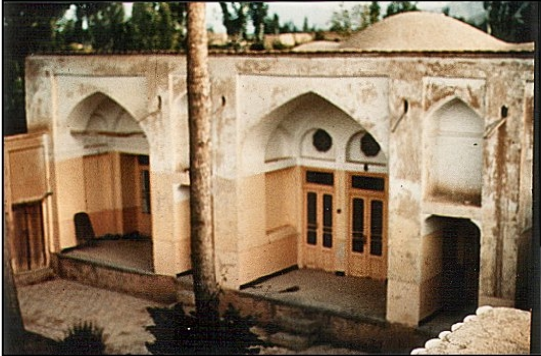
Figure 73: An empty old house in historic citadel of Nain city with its veranda and traditional central courtyard.
