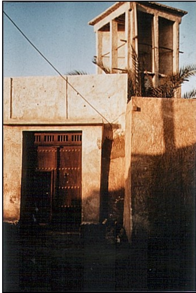
Figure 69: Wind catcher (Badgir), an example of a non-mechanical cooling system.
