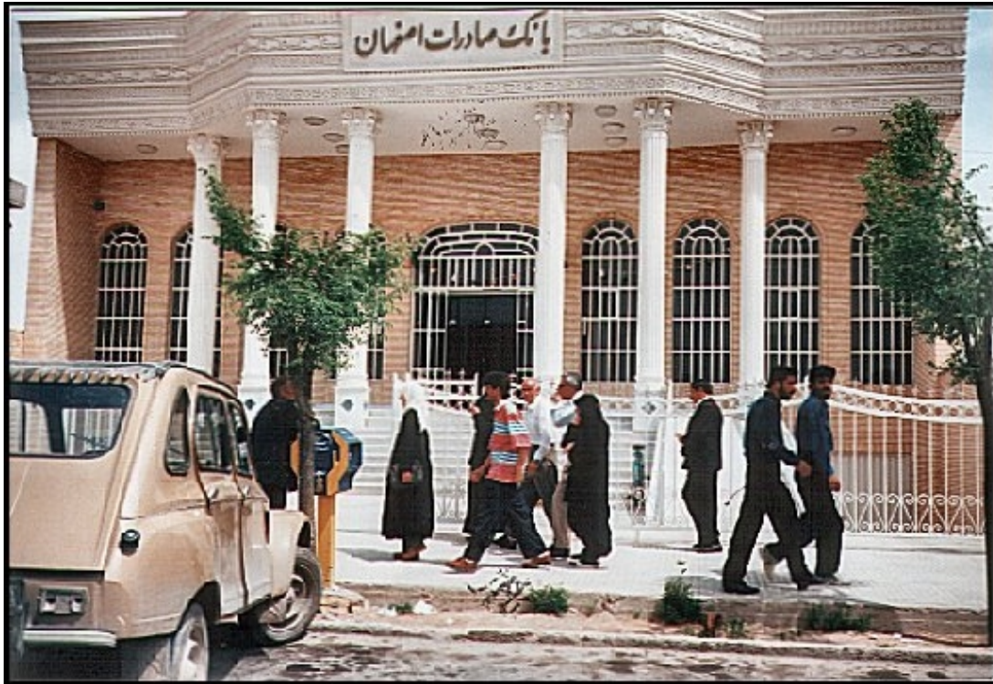
Figure 107: Effect of climatic characteristics on design of modern openings. ‘Saderat Bank’ building in Shahin Shahr new town.
