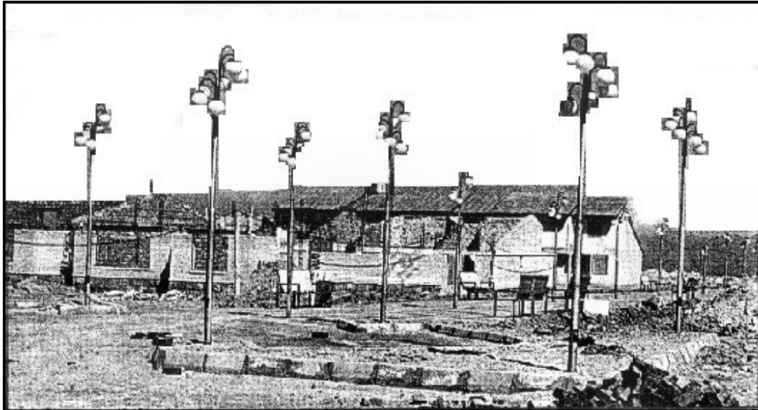
Figure 129: Housing units under construction
