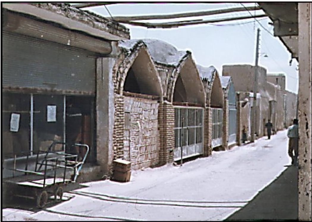
Figure 168: Reconstruction of Neighborhood bazaar with respect to its traditional form in 'Jamaleh' neighborhood in Isfahan city. Source: Author, 1995.
