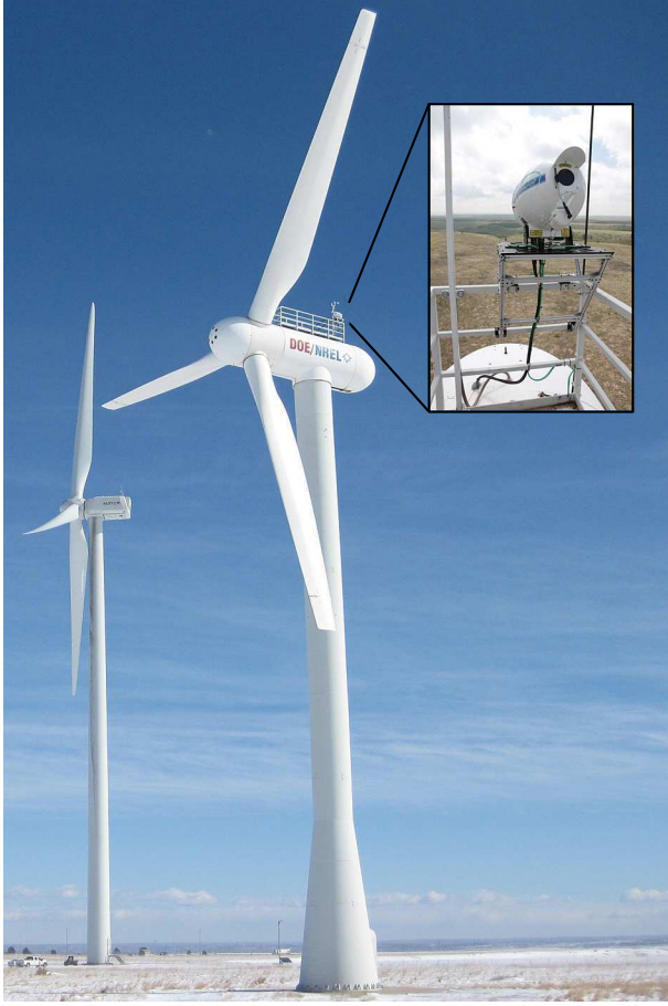
Fig. 1. The OCS installed on the CART3 at the NWTTC.
