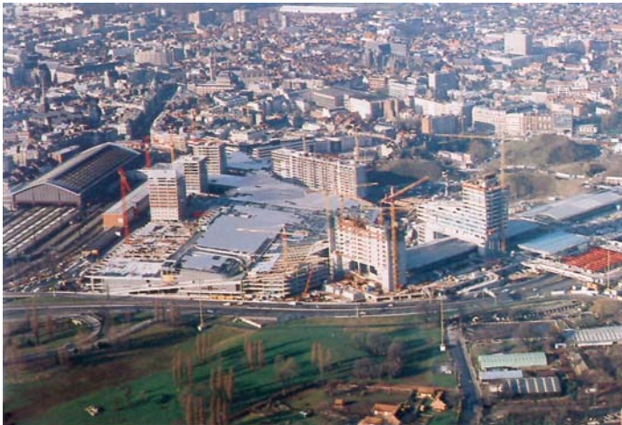
Fig.I. 3: Urban transformation through the HST: The large-scale project "Euralille", literally "built on" the accessibility change by the new HST line London/Paris/Brussels. In the background, the old downtown area of Lille. Source: Ville de Lille 1994, 4
