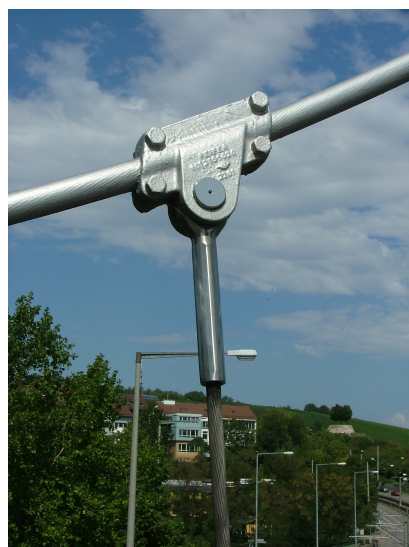
Figure 2: Connector element detail on suspension rope [19]
