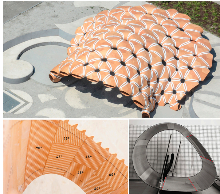
Figure 3. ICD/ITKE Research Pavilion 2015-16: Segmented timber shell and custom lamination of timber veneer to achieve specific bending and strength requirements of architectural shell elements [22].
