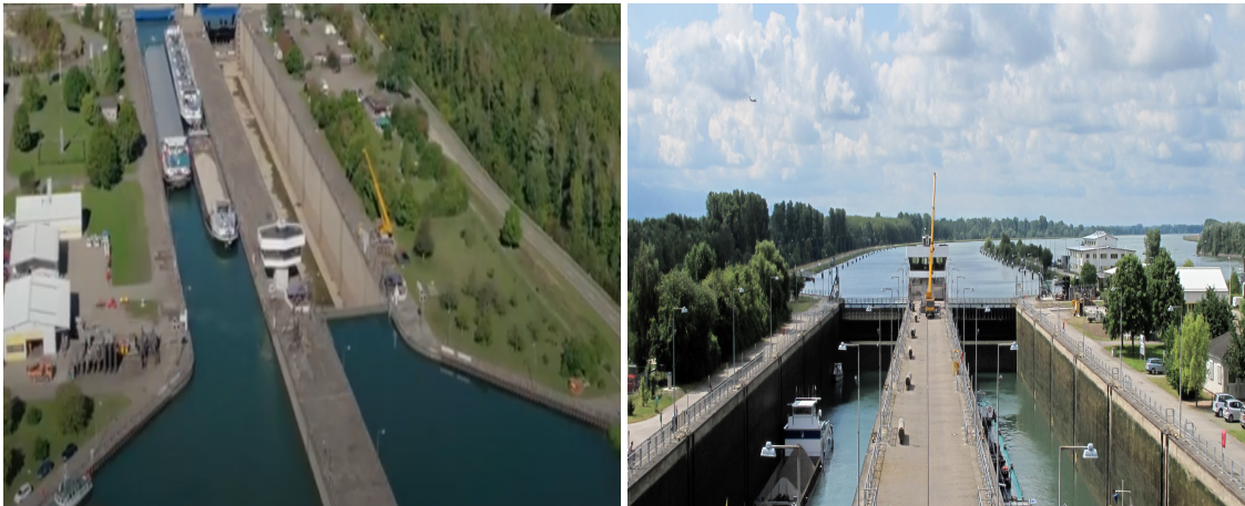
(a) Sluice Iffezheim looking north
