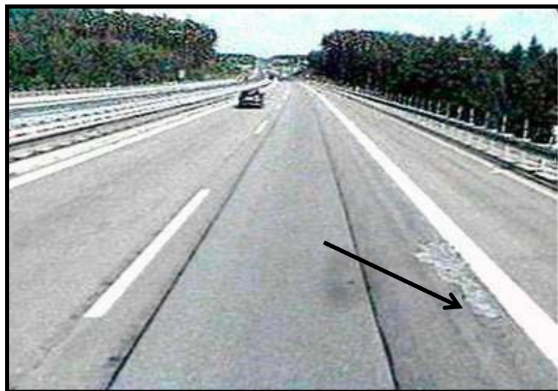
Figure 2.3: Out-breaks (potholes) (FGSV 2006)
