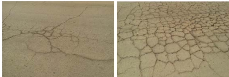
Figure 6.21: Images of this case study: first example of network cracks (block type) (left); second example of network cracks (block type) (right) (UNICOM-UMAP 2014).
