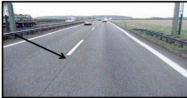
Figure 2.4: Open work seams (FGSV 2006).
