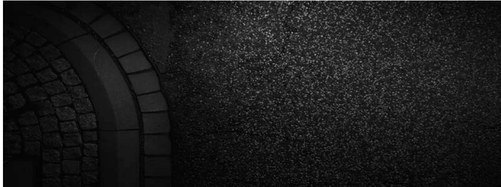
Figure 6.16: Image with high pavement texture and a sidewalk (curb) without cracks (LEHMANN+PARTNER 2014).
