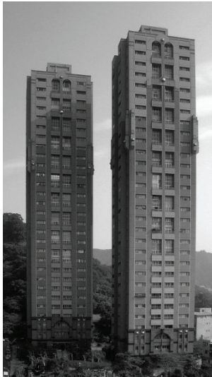
Abb. 184 Cloud Top Buildings ( Yunxiang Building, Dingfeng Building), Taipeh Höhe 135 m, Baujahr 1995
