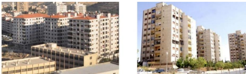
Figure 130 High-rise housing in Aleppo city. Source: The author
