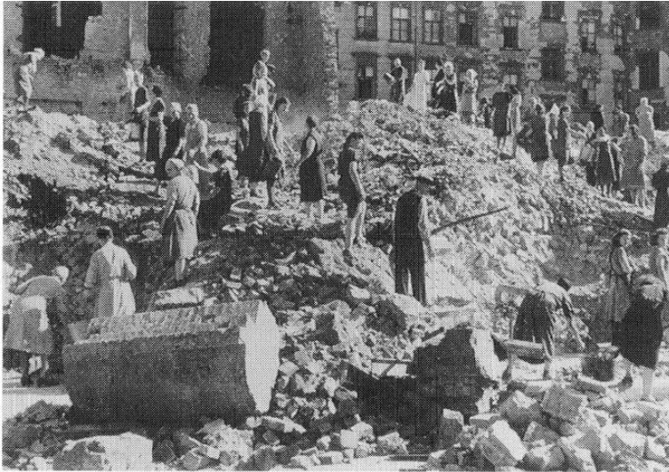
Figure 14: Women in Berlin clearing rubble on the Hagelberger Straße, Kreuzberg, 1949. Source: (Landesbildstelle Berlin, 1 NK, 184 802)
