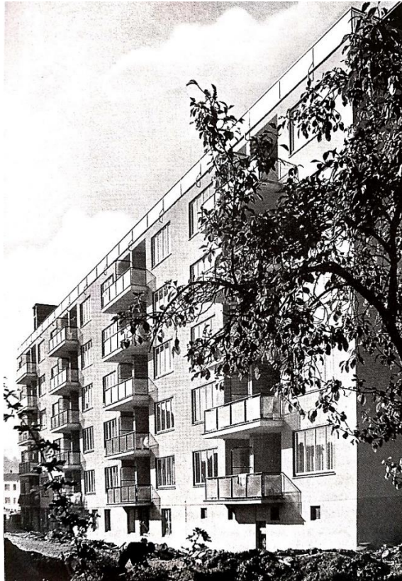
Figure 27 Multi-family houses (Federal employees flats) Reuterstrasse, Bonn 1949-1951, Architekt Max taut. Source: Harlander, 1999
