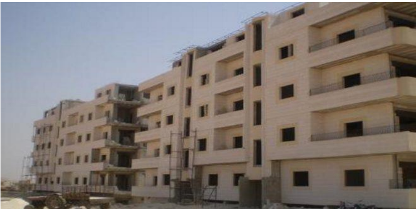
Figure 73 Workers' housing in Syria, Adra near Damascus. Source: Taken by the author
