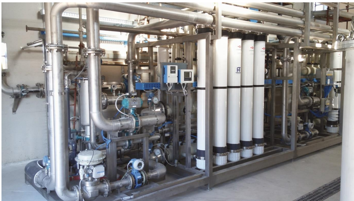
Fig. 1: Capillary ultrafiltration unit
