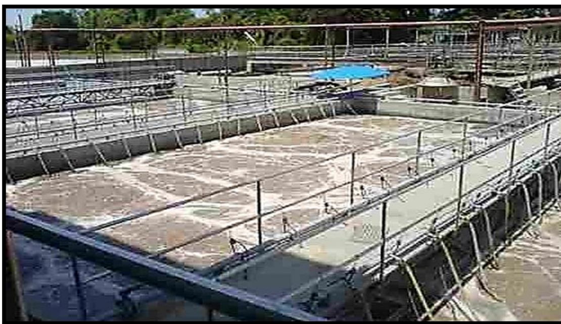
Fig 3: Aeration tanks
