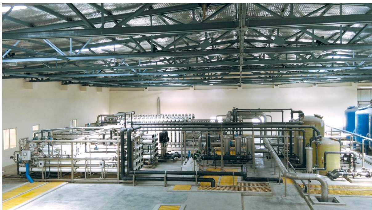
Fig. 2: Three stage reverse osmosis unit
