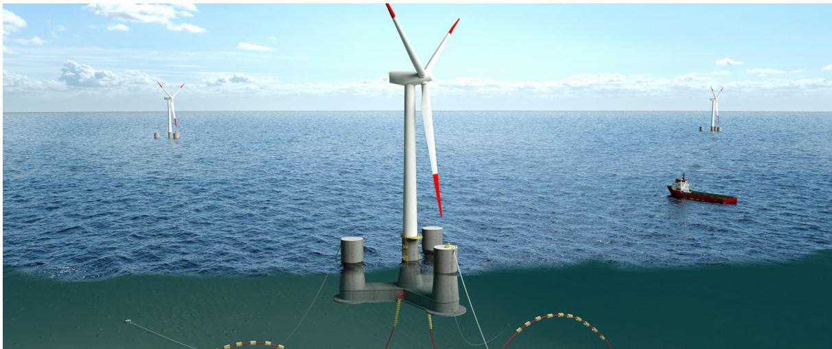
Figure 2: The OO-Star Wind Floater Semi 10 MW concept [1].
