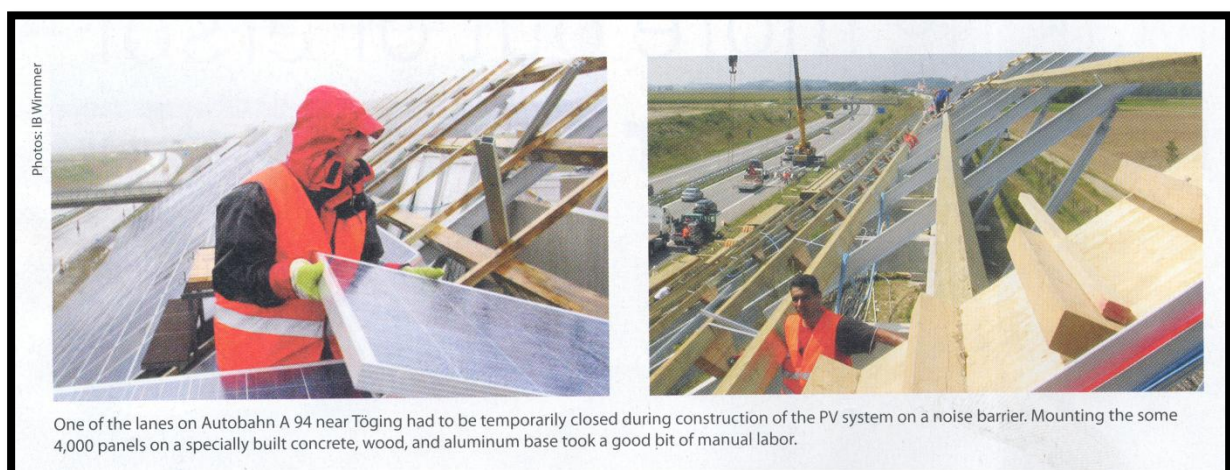
Figure 4-7: INSTALLATION OF PV NOISE BARRIER PILOT SYSTEM IN TÖGING
