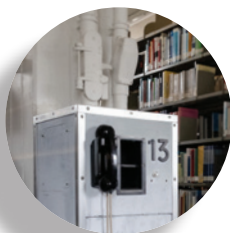
Tube mail station Rohrpoststation
