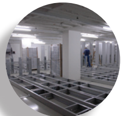
Assembly of the new compact shelves Montage der neuen Kompaktregale
