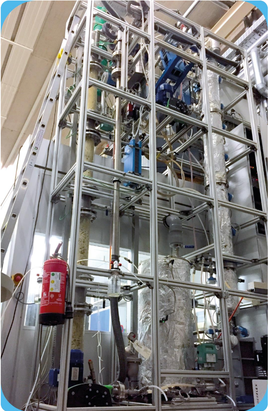
Figure 3-1: Picture of the ABIGAIL pilot plant on the 29.09.2018
