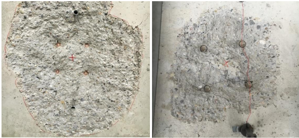
b) c) Figure 8.21. Influence of the crack pattern: a) Load-displacement curves of test series G71-G72; b) failure pattern of test series G71; c) failure pattern of test series G72
