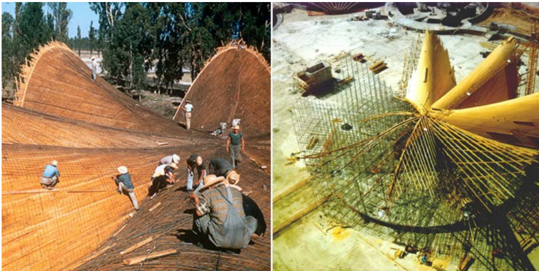
Figure 1.2: Comparison of construction methods. Left: Los Manantiales Restaurant in Xochimilco, Mexico (Guzmán, 1958). Right: L'Oceanogràfic in Valencia, Spain (CMD Ingenieros, 1999).
