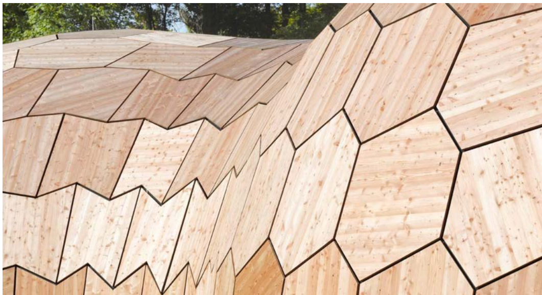
Figure 7.2: Changing plate outlines of the exterior cladding layer reflect the changing curvature of the shell (Halbe, 2014).
