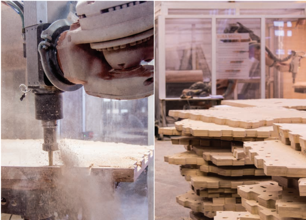
Figure 7.66: Robotic fabrication of plates (Krieg, 2014).
