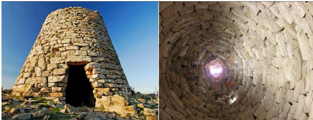
Figure 4.2: Megalithic vaults. Left: The nuraghe Goni, Sardinia. From [36] by Camedda (2008). Right: The corbel vault of the Nuraghe Is Paras. From [42] by Consorzio Turistico dei Laghi (2014).
