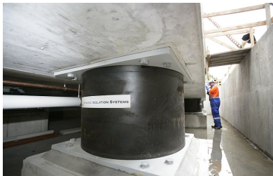
(a) Base isolation system of an electric converter station in New Zealand [33]
