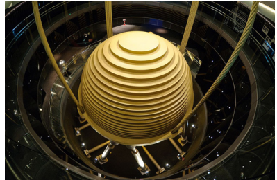
(b) Tuned mass damper installed in the Taipei 101 tower [32]
