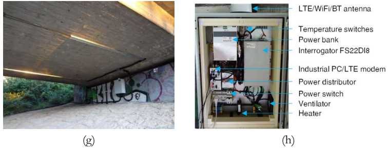
Figure 13. Overview of the bridge and SHM monitoring system: (a) overview of the bridge; (b) MEWP and partial road closure; (c) drilling works for the bracket's fixation; (d) view of the quasi-distributed sensor's lines; (e) view of installed sensors; (f) an LGFBG sensor with 2.05 m gauge; (g) view of the cabinet control installations; (h) detailed view inside the cabinet control.
