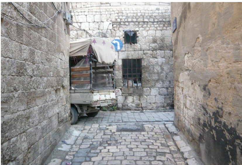
Fig. 3- 23 Delivery cars driving produce fumes, cause vibrations and threaten the physical structure of buildings aligning the narrow medina streets
