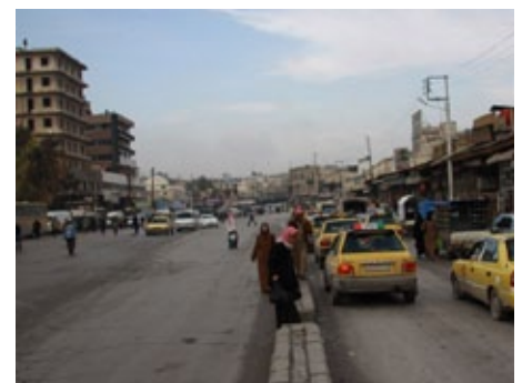
Fig. 3- 62 Absence of any light-controlled or marked crosswalks for pedestrians on Antakia Street, and the median is too narrow and high
