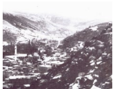
Fig. 4- 3 Settling the valley along the water source (source: courtesy of GAM)
