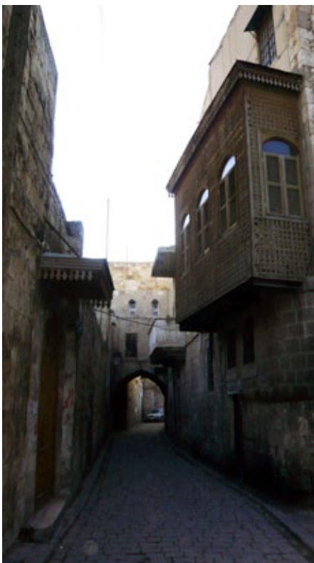
Fig. 3- 50 & 3- 51 Bab Qinnisreen before and after rehabilitation (source of 2- 45: RehabiMed)
