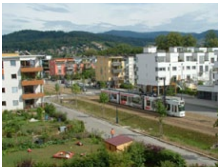
Fig. 2- 50 A tram line passes along the main axis of the Vauban residential district (source: Melia 2006)
