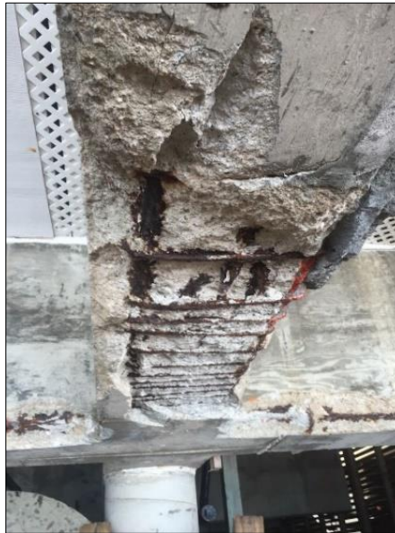
Figure 2-15. Explosive spalling on a concrete structural member (Source: see bibliography).
