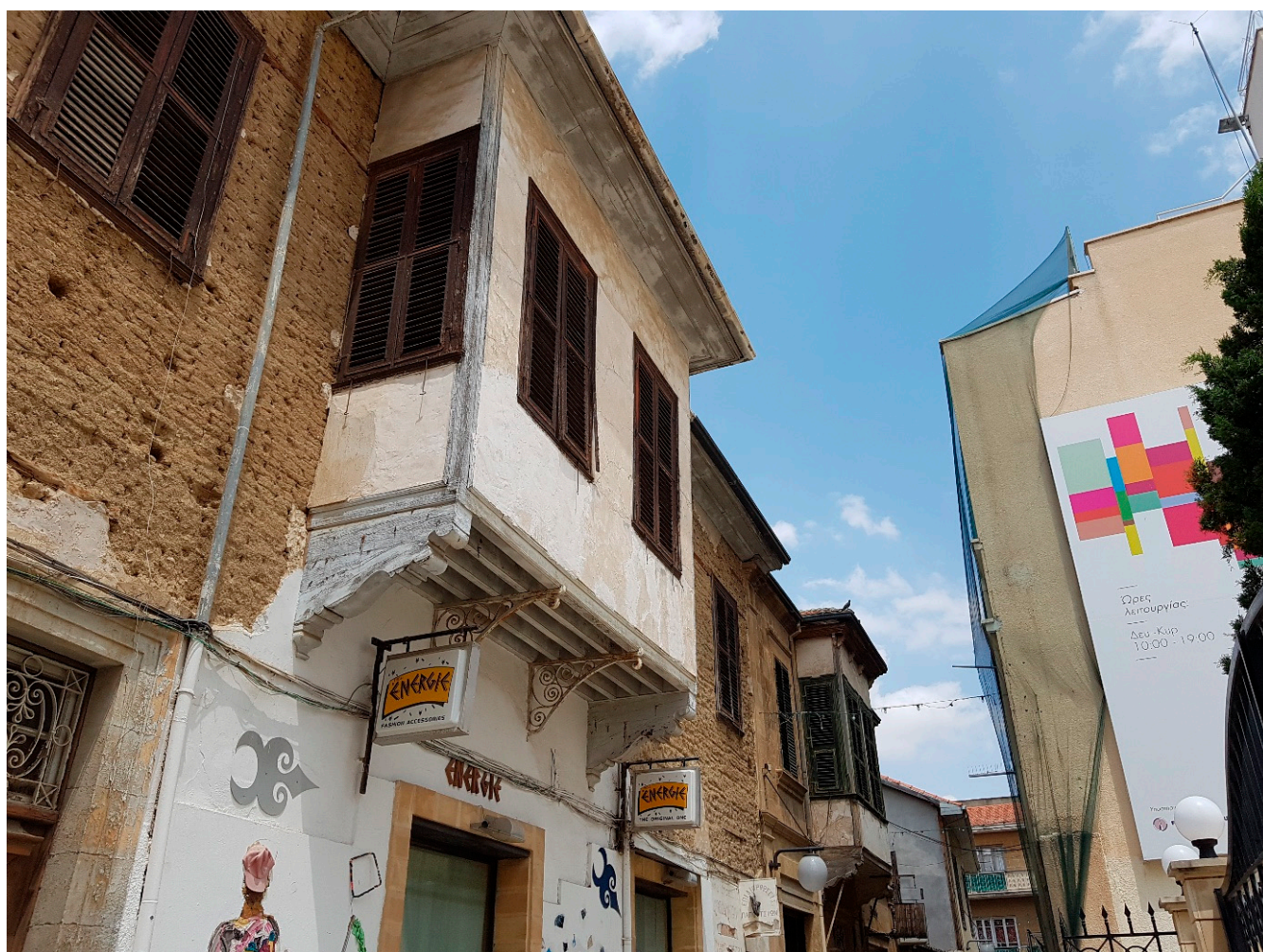
Figure 18. Kishk, the cantilevered space typical of Turkish houses, with transformable shutters with hygroscopic performance, Nicosia, Cyprus (photo: Davidová, 2018).
