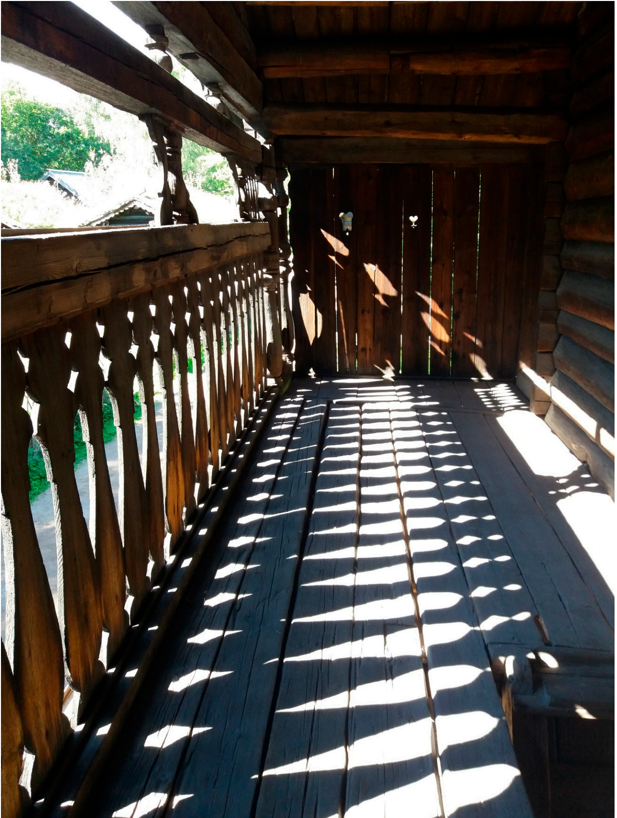
Figure 24. Breathing screen on a svalgang of a store house from Nes in Hallingdal, dated 1700–1797, now in Oslo’s Open Air Museum (photo: Raková 2017—published with the permission of Raková).
