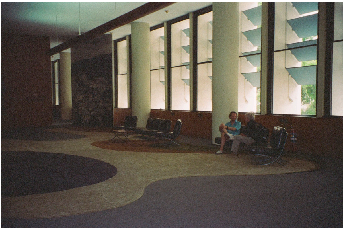
Figure 14. Le Corbusier, Lucio Costa, et al., Ministry of Education and Health, Rio de Janeiro, 1937–1942, operable outdoor jalousie, ‘brise-soleil’ (photography: Davidová, 2005).
