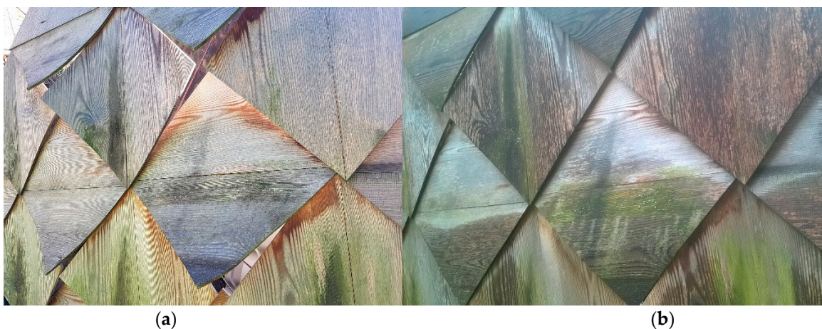
Figure 38. Ray 2 prototype from left to right: (a) in semi-dry June 2018 weather when the screen is open for boundary exchanges between exterior and semi-interior; (b) after light rain in April 2017 when the system is closed, which does not allow the humid or cold air to pass through the boundary, after five and four years, respectively, of exposure to weather and biotic conditions (Photos: Davidová, 2017–2018).
