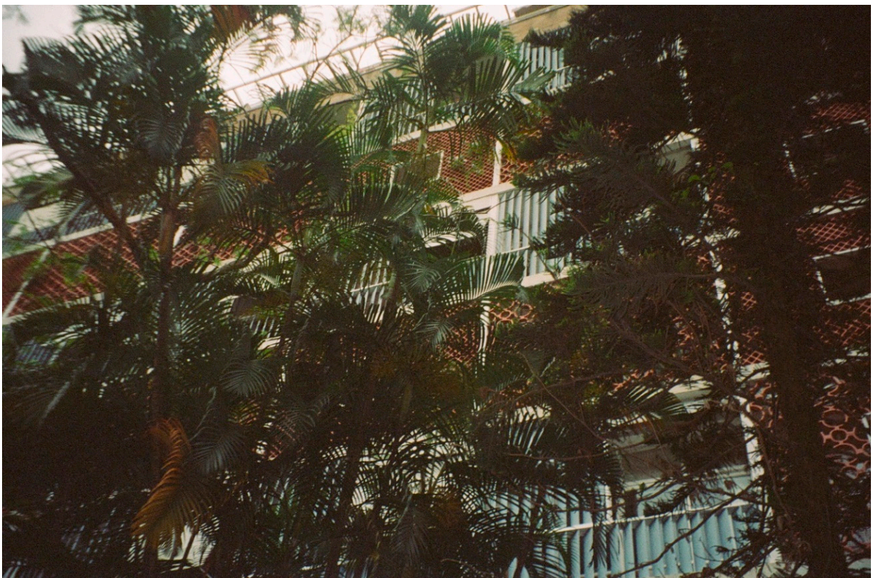
Figure 12. Costa, Parque Guinle, Rio de Janeiro, 1947–1953, combination of cobogós, an operable 'brise-soleil' moderating a microclimate, and letting vegetation grow into semi-interior spaces of an apartment block (photo: Davidová, 2005).
