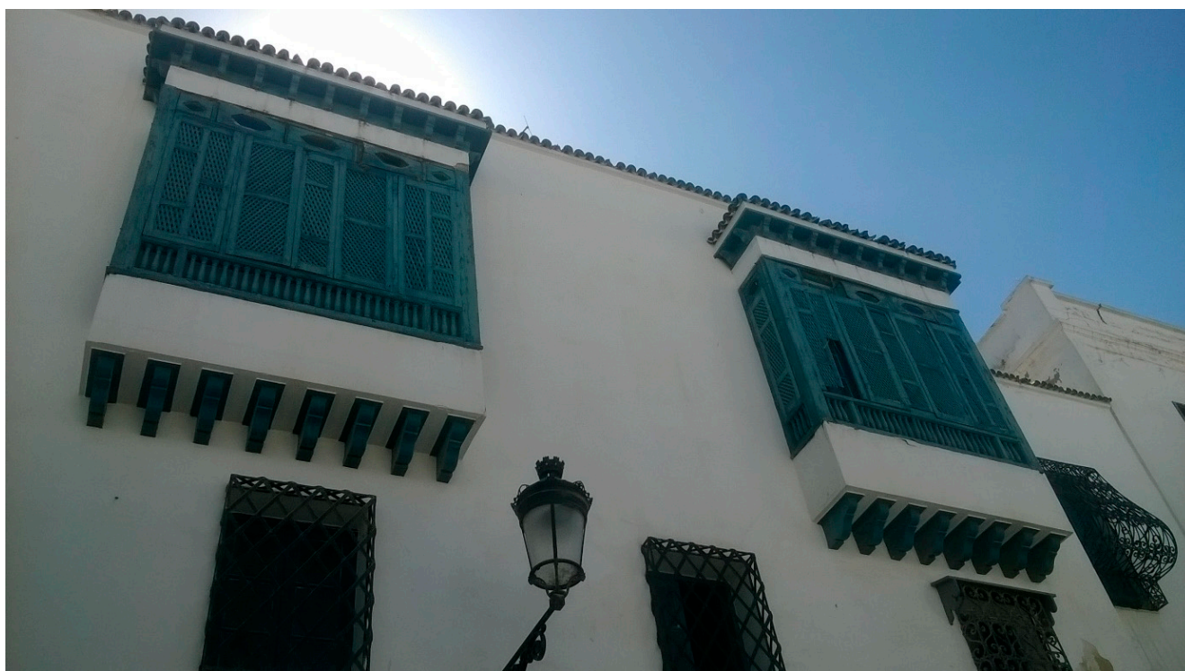
Figure 20. Kishk is a cantilevered space typical for a ‘Turkish House’ that is often enveloped by mashrabīya [37] in Mediterranean climate of Tunis (photo: Davidová, 2017).
