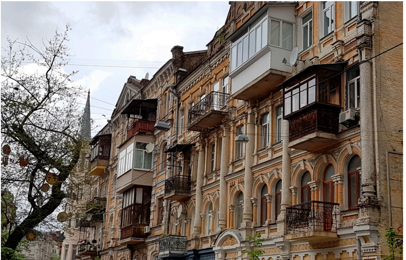
Figure 28. Kyiv, vernacular add-on spaces built on the basis of former balconies (photo: Davidová, 2018).
