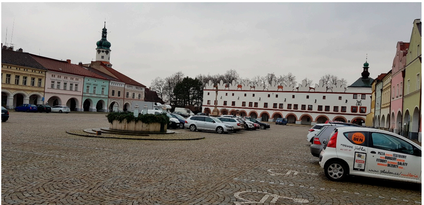
Figure 1. Semi-interior arcade spaces of a renaissance square in Nové Město Nad Metují, Czechia. These spaces have been largely inhabited by swallows. The human citizens believe the swallows bring them luck. They also lower the number of mosquitoes and are a sign of healthy environment (photo: Davidová, 2021).
