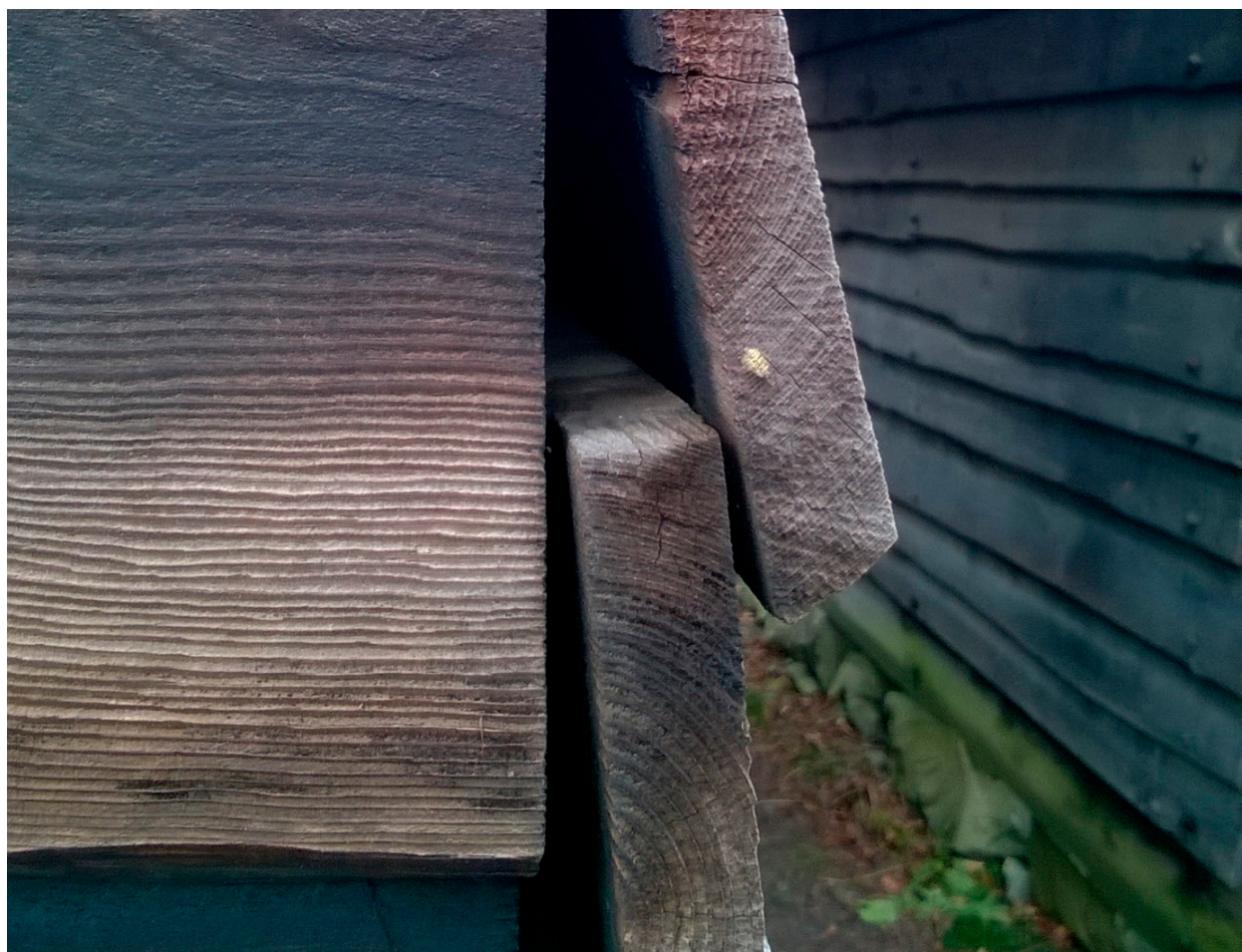
Figure 26. Breathing envelope that uses material performance of warping due to hygroscopicity of a store house from Nes, Øvre Valdsaroy, now in Open Air Museum in Oslo (photo: Davidová, 2016).
