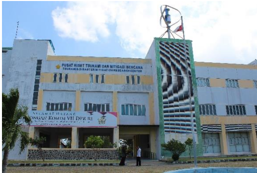
Figure 58. Escape building Banda Aceh. Source: Lucas, 2016.
