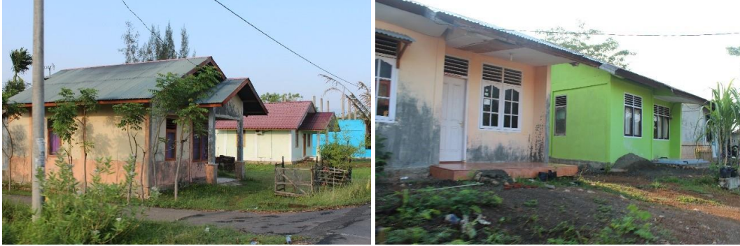
Figure 66a-b. Lambung village, Banda Aceh. Source: Lucas, 2016.
