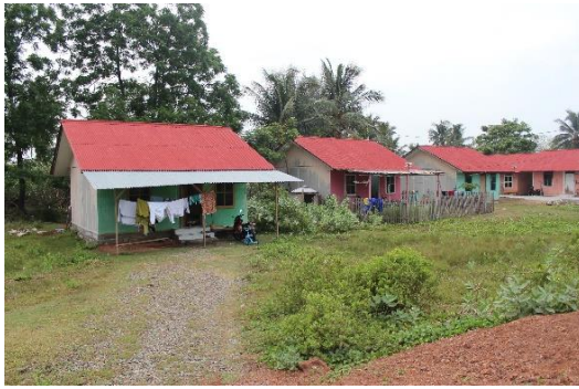
Figure 56. Settlement with panels containing asbestos, Banda Aceh. Source: Lucas, 2016.
