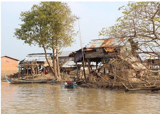
Figure 35. Stilt house in Cambodia after a storm I. Source: Lucas, 2013.
