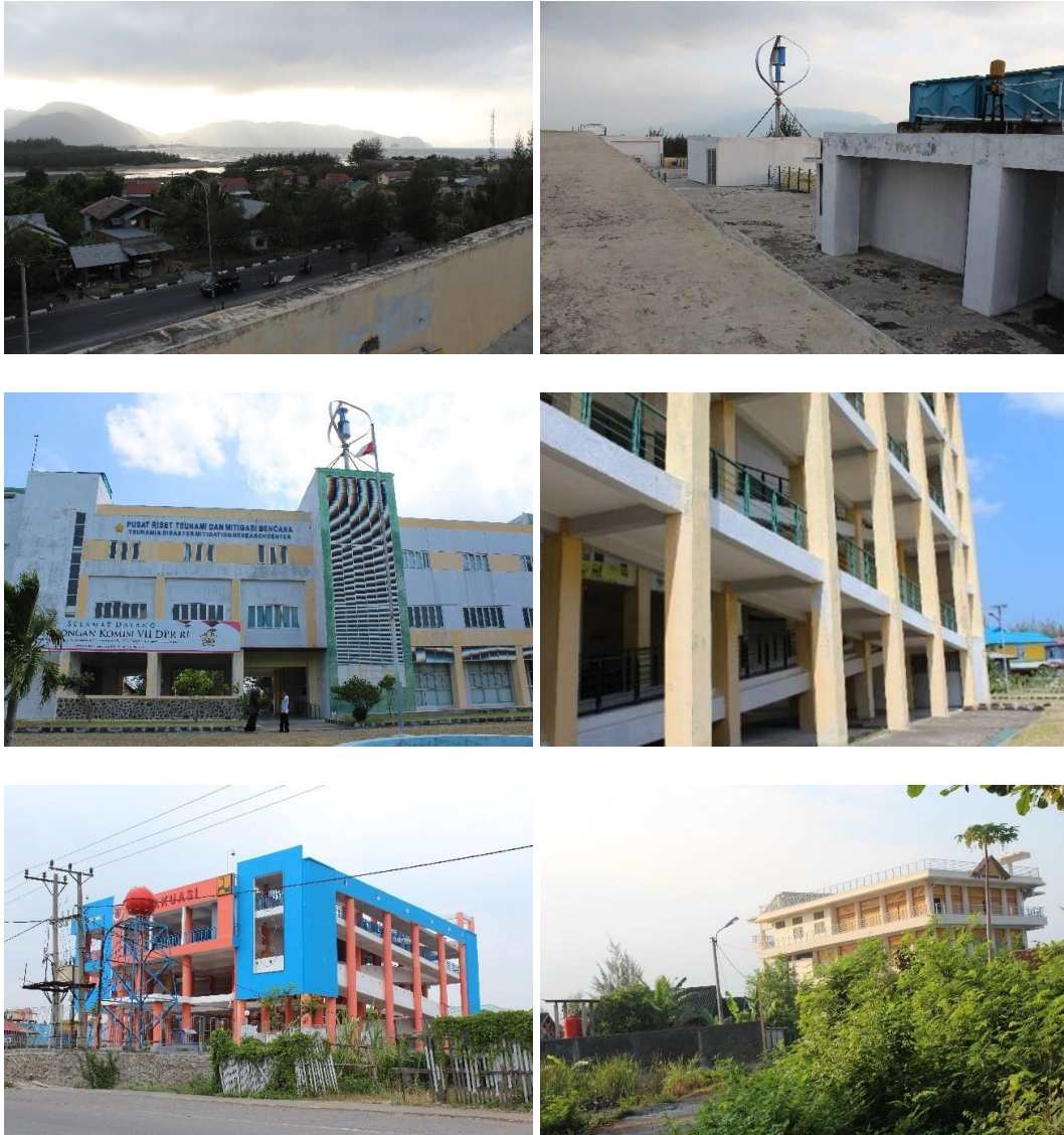
Figure 72a-f. Escape buildings Banda Aceh. Source: Lucas, 2016.
