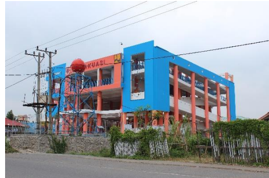
Figure 59. Escape building Banda Aceh. Source: Lucas, 2016.
