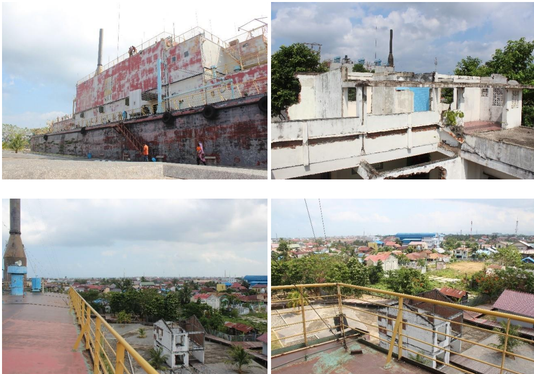
Figure 79a-c. PLTD Apung 1, an electricity-generating vessel weighing 2600 tonnes, carried about 3 km inland by the tsunami 2004, Banda Aceh. Source: Lucas, 2016.
