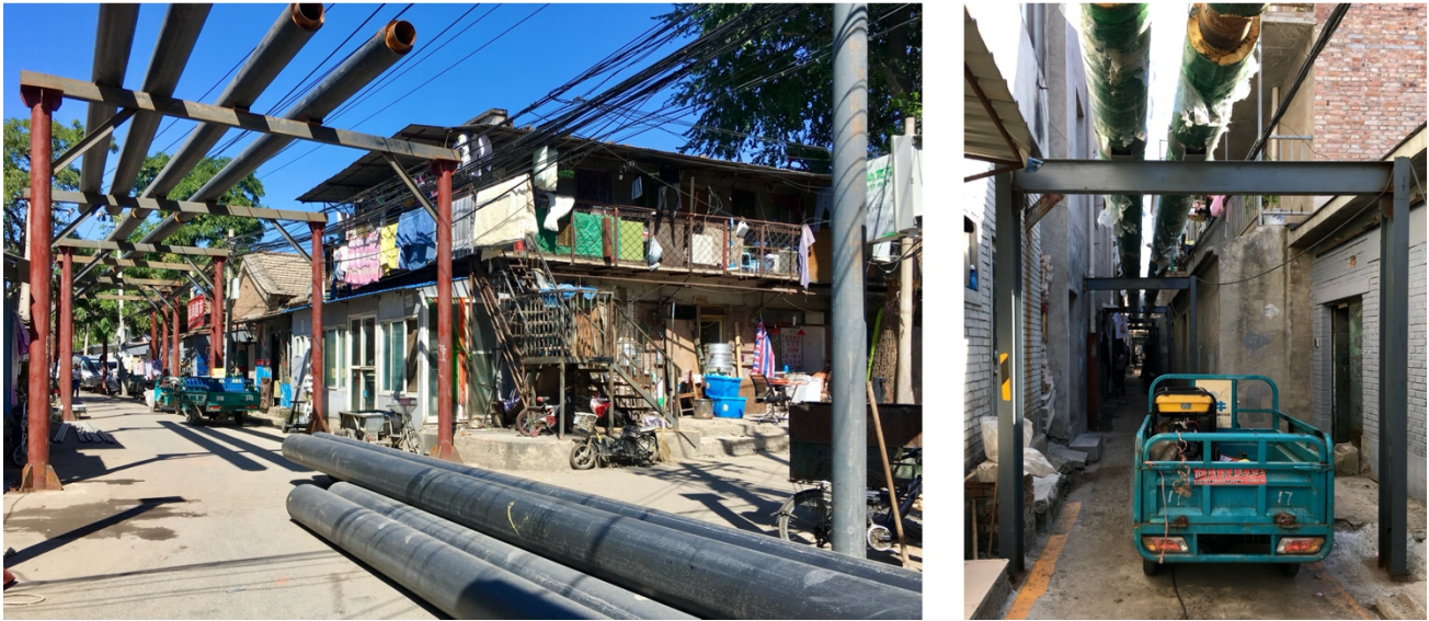
Figure 6: Ongoing ‘coal to gas’ project in Xishan village and Yuanmingyuan East Street in Haidian District. Source: Author, September 2017.
