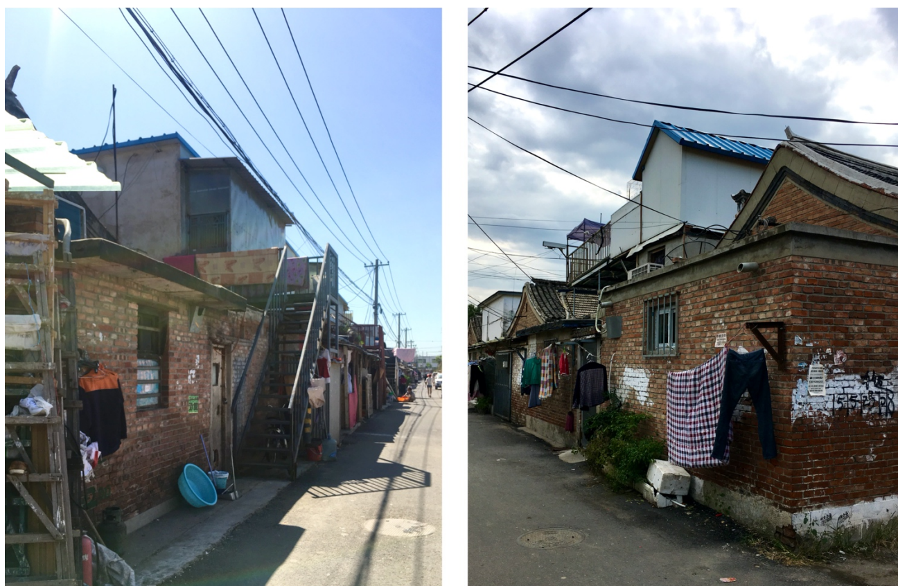
Figure 14: Vertical extensions on top of the original buildings with external staircases in Shigezhuang. Source: Author, September 2017.
