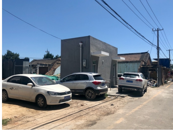
Figure 11: The grey building in the middle is the government-funded public toilet, which remained clean both outside and in, while the surrounding houses were emptied and partially demolished and the site was turned into a parking lot. Source: Author, July 2019.
