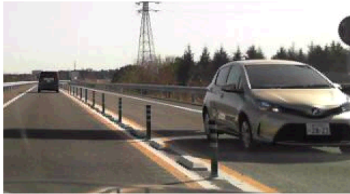
Figure 6.10: Poles and stone blocks separating opposite sides of traffic. Image: Valeo.
