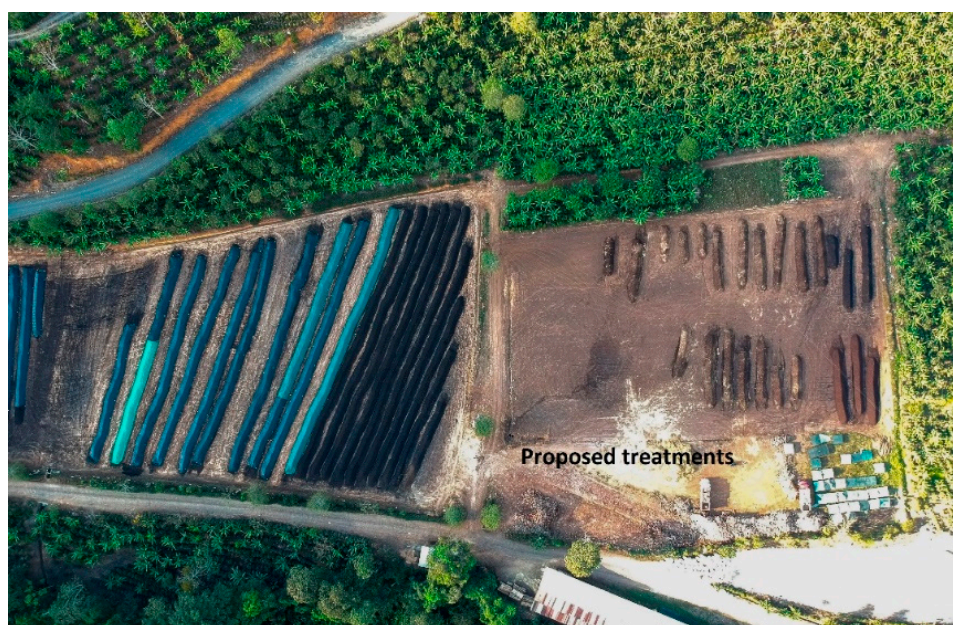
Figure 1. Aerial photo of the proposed treatments T1–5 (right section) and aerial photo of the current treatment at the mill TC (left section).
