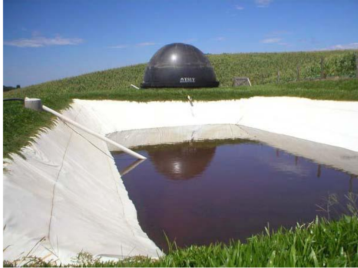
Figure 5-16 Lagoon biogas plant for pig industry in Brazil (Henn, 2005)
