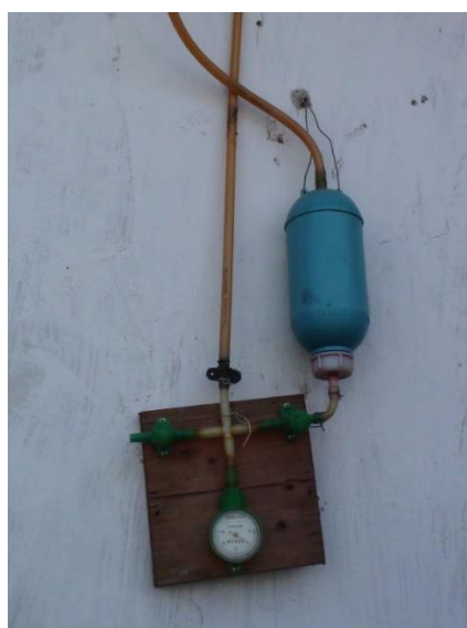
Figure 4-7 Household biogas digester in China – measurement of gas pressure
