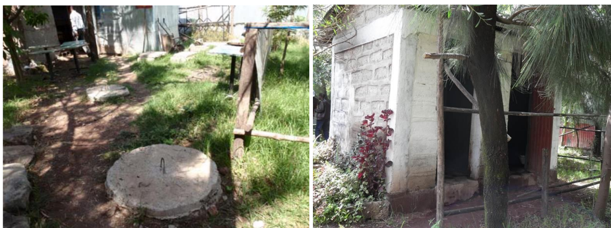
Figure 5-6 Biolatrine in Addis Abeba (ENDA, 2009)
