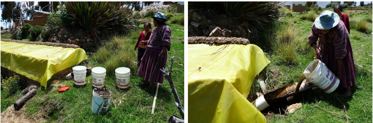
Figure 5-11 Inlet process of biogas digester in Bolivia (Martí-Herrero, 2010)
