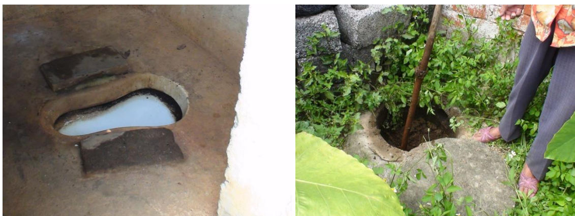
Figure 4-5 Household biogas digester in China - Inlet from toilet waste (right) and cow manure (left)
