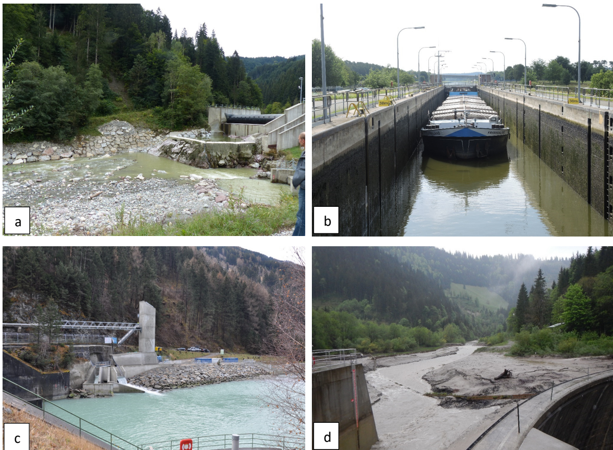
Fig. 8: Different kind of disturbances of the continuity of the watercourse as result of the construction of reservoirs (a) diversion hydropower plant in the Austrian Alps; (b) lock Eckersmühlen at the Main-Donau-waterway, Germany; (c) technical fish elevator at the weir Runserau, Austria; (d) sedimentation in a small reservoir in the Austrian Alps.
