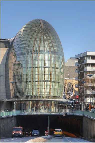
FIG. 1.5: Shading system inside the double-curved façade of the Peek & Cloppenburg Flagship store Cologne. (Photo by © Raimond Spekking / CC BY-SA 3.0 (via Wikimedia Commons))
