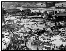
Figure 1.2: Three different historical disasters initiated by cracks. On the left the Boston Molasses Disaster from 1919 where a large tank burst is shown. In the middle a picture of the hull fracture of the SS Schenectady from 1943 is given. On the right a crack in the hull of a de Havilland Comet aircraft is shown. This failure led to several plane crashes in the 1950s.
