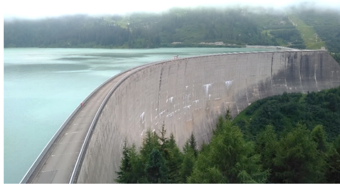
Figure 6.26 Side view of the arch dam Kops in August 2019
