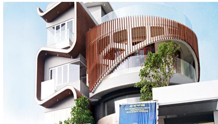
Figure B3-16. Resysta® being applied in a building façade by the Asian architect: Nguyen Lam Dien in Vietnam, (Resysta International GmbH).
