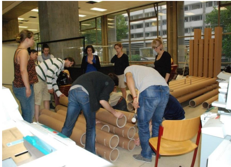
4-Preparing the other wall separately before fixing it to the finished parts of the pavilion
