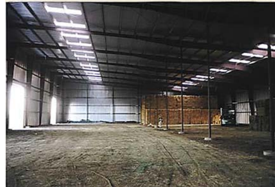
Figure B1- 9. Different storing systems (Huisman, et al., 2002). Up: Pole barn storage, Down: Metal building for closed storage
