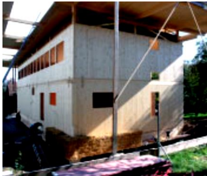
(a): The stacking process of the bales before plastering- (bmvit- Austrian Federal Ministry for Transport, Innovation and Technology, 2005)
