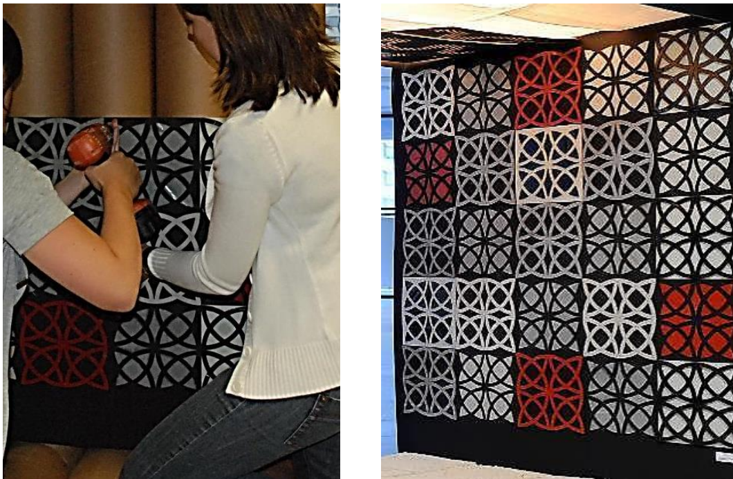
Figure D 3-9. Illustration of the BiOnament designed green biocomposite panel, applied as an architectural screen within the constructed pavilion: Eco-Pavilion (see Appendix). Photo credit: Left: Dahy,H.; Right: Miklautsch,B.
