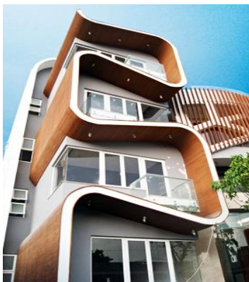
Figure B3-16. Resysta® being applied in a building façade by the Asian architect: Nguyen Lam Dien in Vietnam, (Resysta International GmbH).
