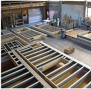
Prefabrication process taking place prior to straw bale filled studs installations.
