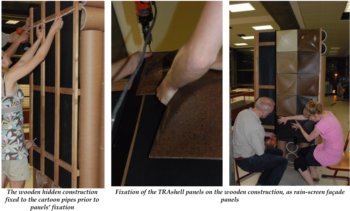
Figure X-9. Illustration of the TRAshell panels' fixation on the Eco-Pavilion's exterior elevation as a façade rain-screen application.
