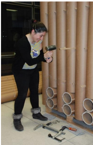
5-Digging in the wood connectors
