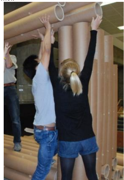
6-Balancing the elevated sides before hand-lifting the ceiling
