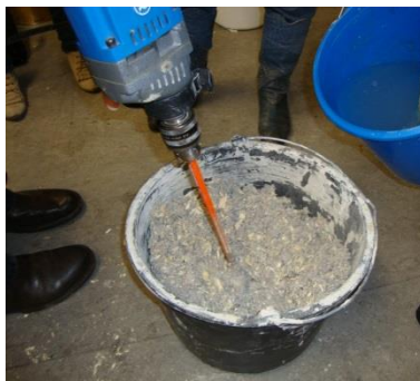
1- Mixing the fibrils with the glue
