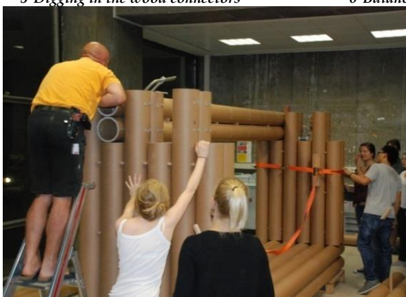
7-Fixing the ceiling to the structure to the body
