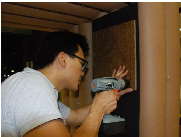
Screwing the STRAWAVE panels after drilling them
