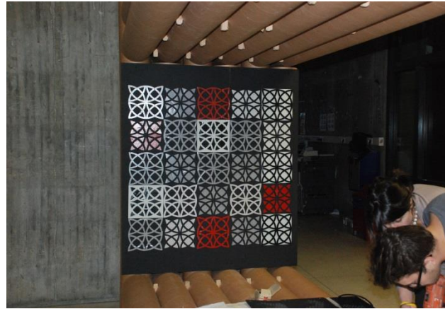
BiOrnament panels fixed as inner cladding system
