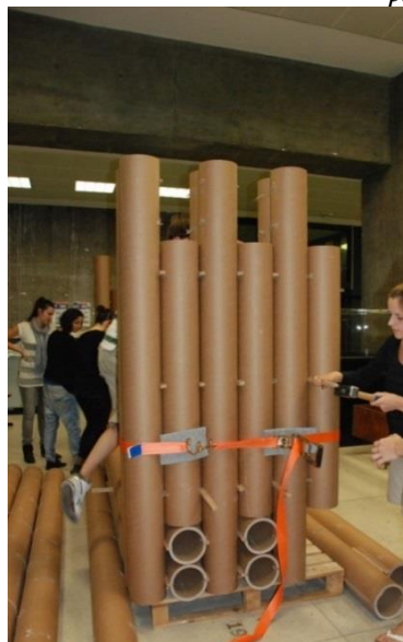
6-Balancing the elevated sides before hand-lifting the ceiling
