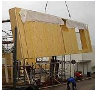
Installation using a crane
