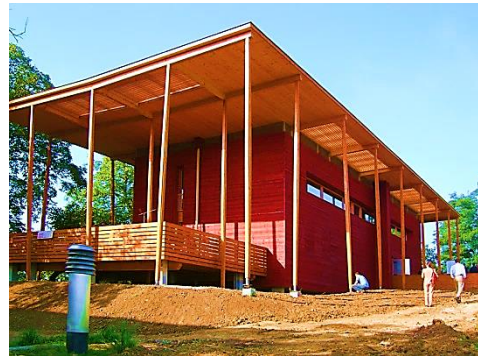
(b): The finished S-House building at its final stage- (Unser Strohhaus Bau GmbH)
