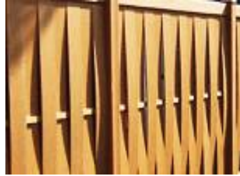
Figure B3-15. TerraWeave™ of recycled HDPE and straw, forming 3D-formed screen, (Natures Composites TM- organic building products, 2011).
