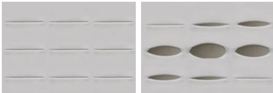
Figure 5 – Textile building envelope with integrated pneumatic apertures for controlled ventilation of interstitial membrane spaces (© ILEK Uni Stuttgart, 2011)
