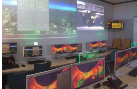
(b) IRS Control Room
