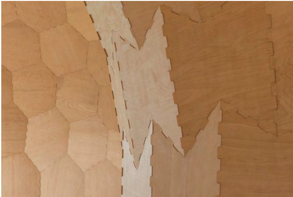
Figure 7.60: Photograph of concave plates with finger joint connections. The finger joints at the edges that form a negative polygonal angle are facing inwards (Image by ICD/ITKE/IIGS University of Stuttgart).
