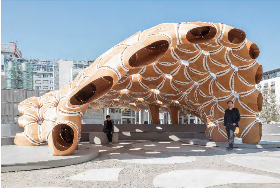
Figure 7.51: The ICD/ITKE Research Pavilion 2015-16. Image by ICD/ITKE University of Stuttgart.
