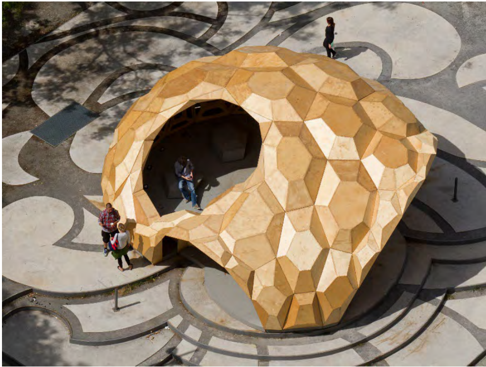
Figure 7.9: The ICD/ITKE Research Pavilion 2011 (Image by ICD/ITKE University of Stuttgart).
