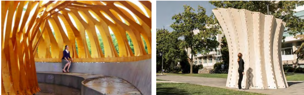
Figure 5.3: Left: the elastically bent plywood strips of the ICD/ITKE Research Pavilion 2010 (Image by ICD/ITKE University of Stuttgart). Right: elastically bent and interconnected plywood strips make up the double-layered structure of a segmented shell prototype (Image by ICD University of Stuttgart).
