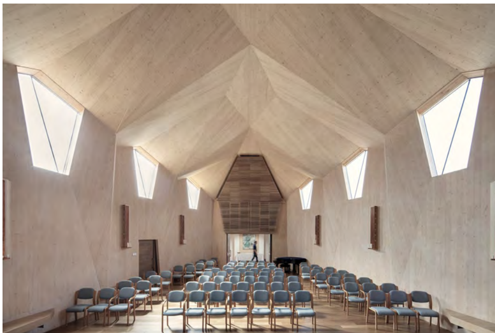
Figure 4.3: Vaulted CLT church in Stroud by Nicolas Pople Architects (Image by Fernando Manoso Borgas).
