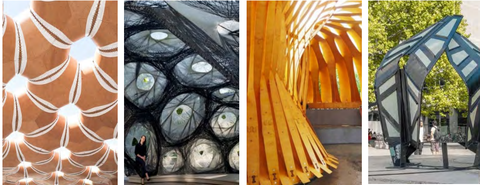
Figure 3.1: Examples of the transfer of biomimetic principles to architectural design research. From left to right: (1) gradual morphological variation in building elements (Image by ICD/ITKE University of Stuttgart); (2) multi-scalar variation of form through fiber placement in building modules (Image by ICD/ITKE University of Stuttgart); (3) anisotropic arrangement and performance of building elements (Image by ICD/ITKE University of Stuttgart); (4) multifunctional building elements through variation in material for kinetic structures (Image by ICD/ITKE/ITFT University of Stuttgart).
