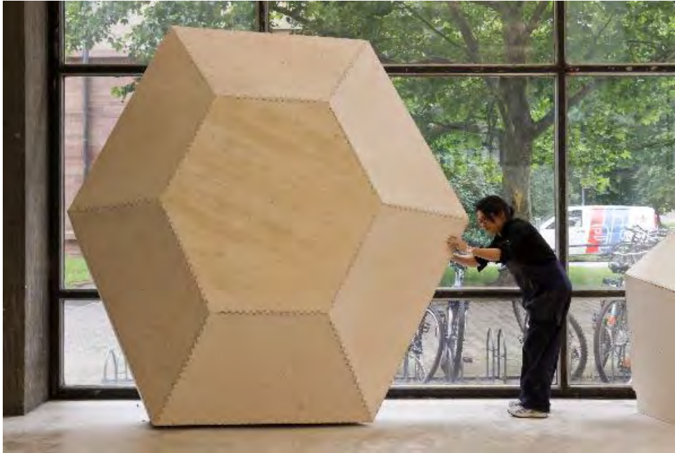
Figure 7.6: The building system exhibits two hierarchies of building elements (individual plates) and building components (modules made from 12 to 21 plates) (Image by ICD/ITKE University of Stuttgart).
