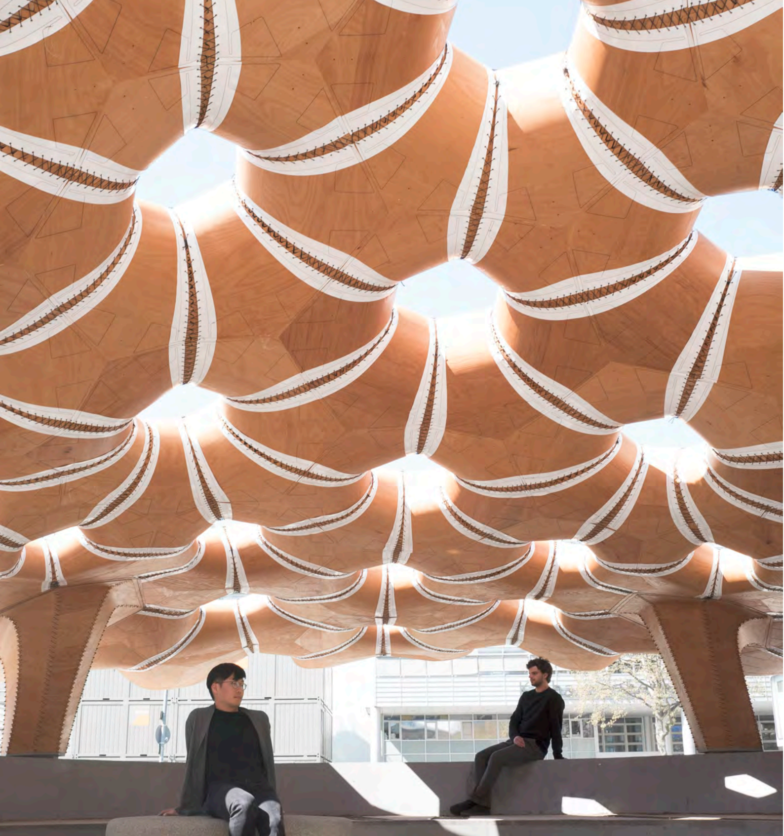
Figure 7.45: The ICD/ITKE Research Pavilion 2015-16 (Image by ICD/ITKE University of Stuttgart).
