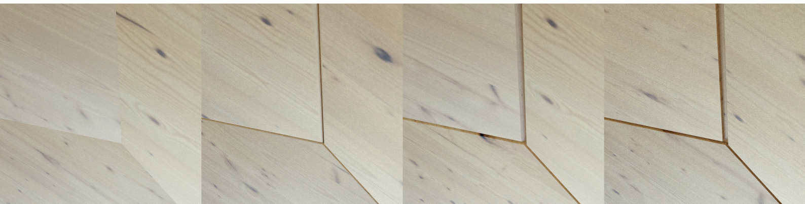
Figure 5.31: Joint details: butt joint (left), rounded edge (center left), 45° chamfer (center right), and straight shadow gap (right).
