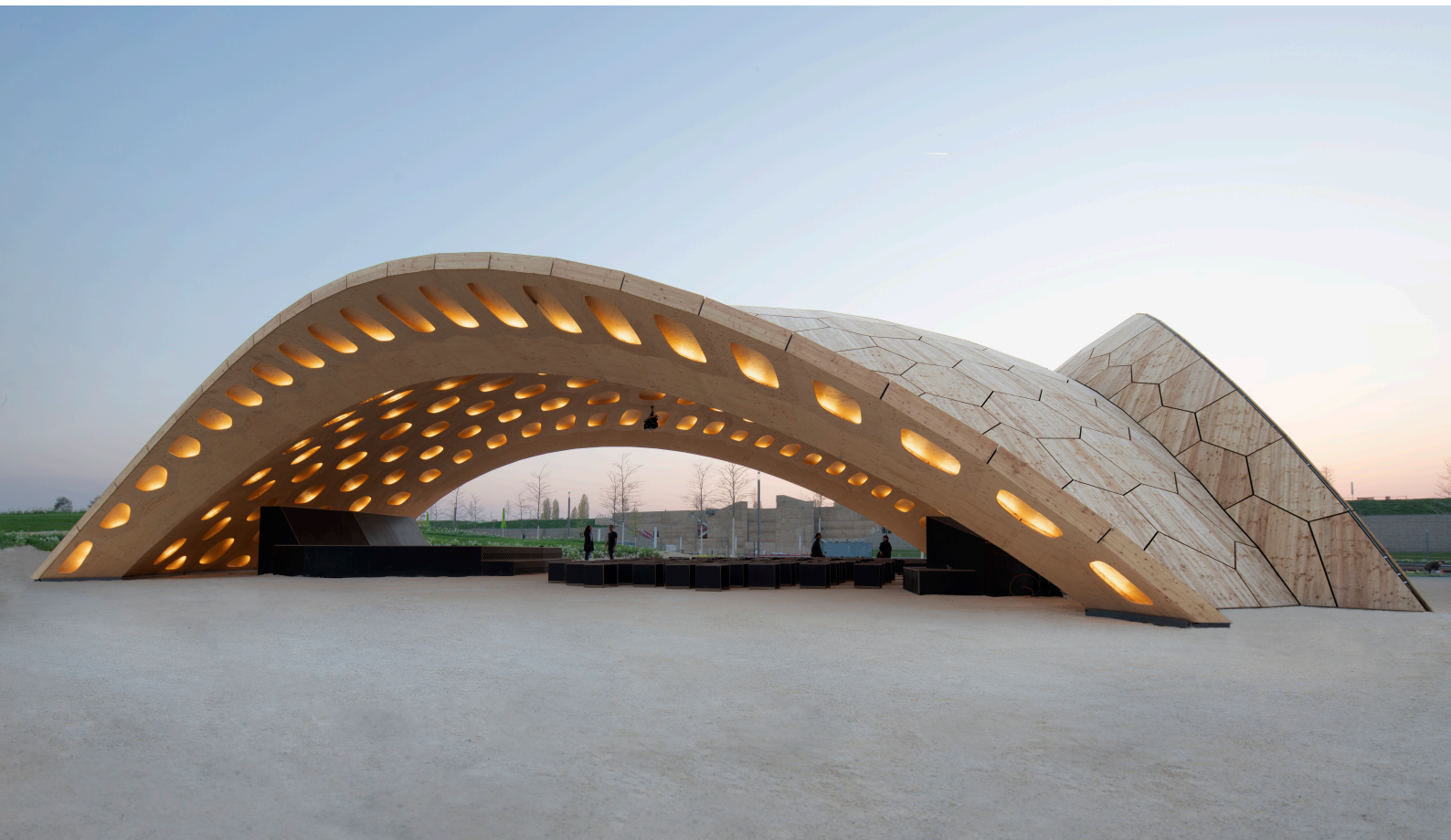
Figure A.6: The BUGA Wood Pavilion. Image source: ICD/ITKE, University of Stuttgart
