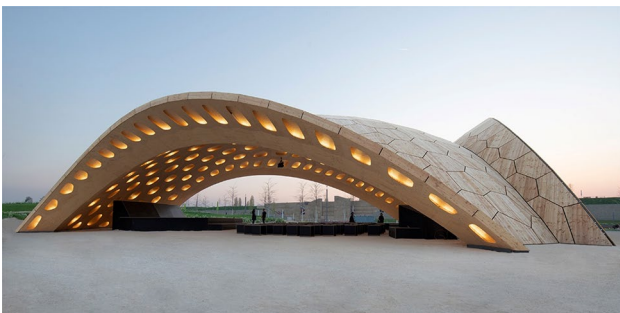
Fig. 1 The BUGA Wood Pavilion spans 30 m over a central event area on the ‘summer island’ in Heilbronn
