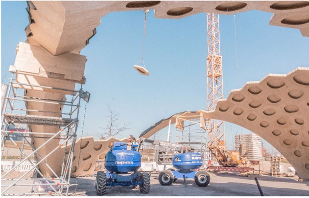
Fig. 14 Due to detailed sequencing, no sorting was necessary on site. Each cassettes were iteratively taken off the stacks and directly mounted in the shell
