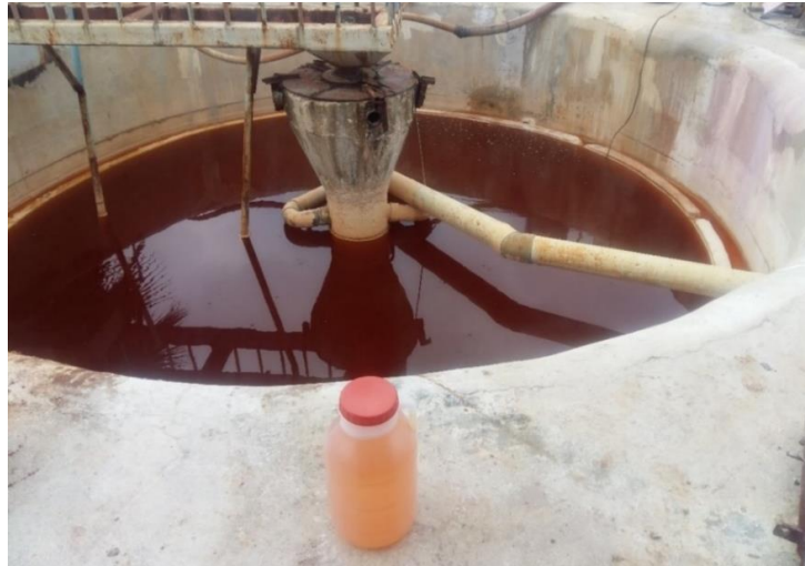
Fig. 27 Sedimentation basin before adding chlorine in the Acryl Tab company (photo: E. Khalilzadeh Shirazi)
