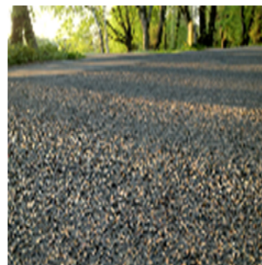
(b) Asphalt Surface
