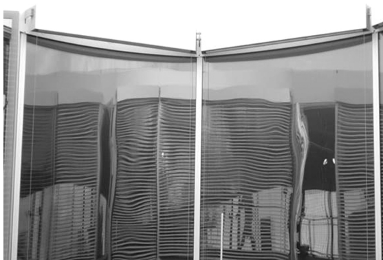
Figure 2.6.: Optical distortion of a single curved, thermally bent insulating glass unit.
