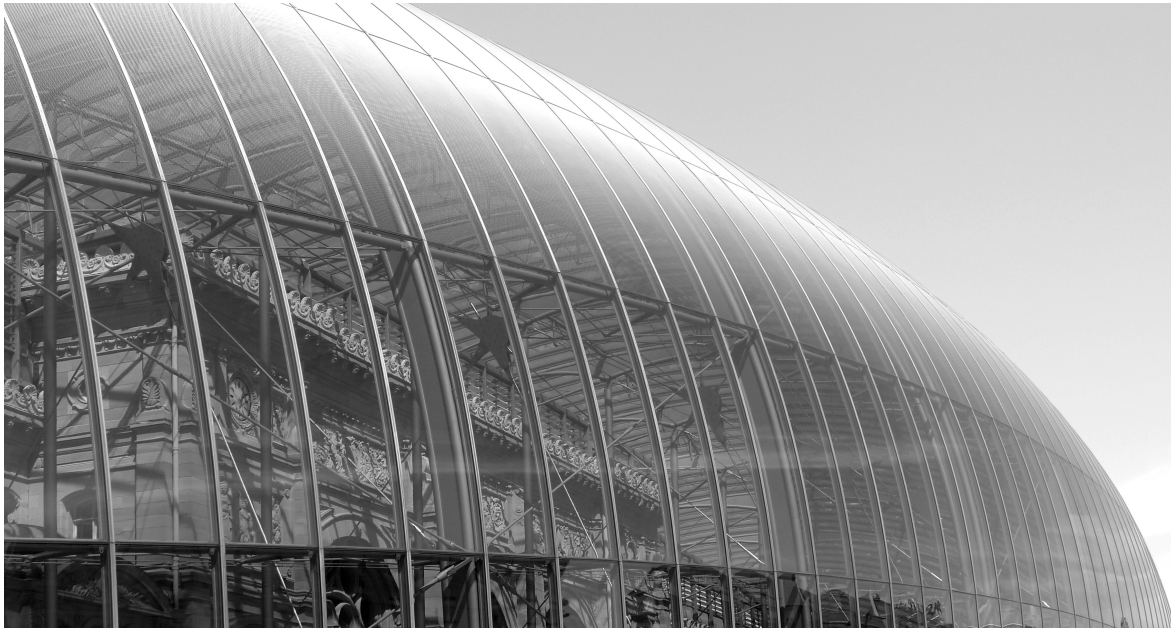
Figure 1.6.: Cold bent glass façade of Strasbourg Central Station.
