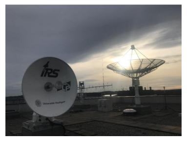
Figure 5-19: Two ground stations at IRS of the University of Stuttgart. On the left: the 2.5 m S-band ground station which is used for the current satellite mission. On the right: the new 4.5 m ground station developed and built for the ROMEO mission with the parameters of Table 3-2. The STR and MAL ground station are identical
