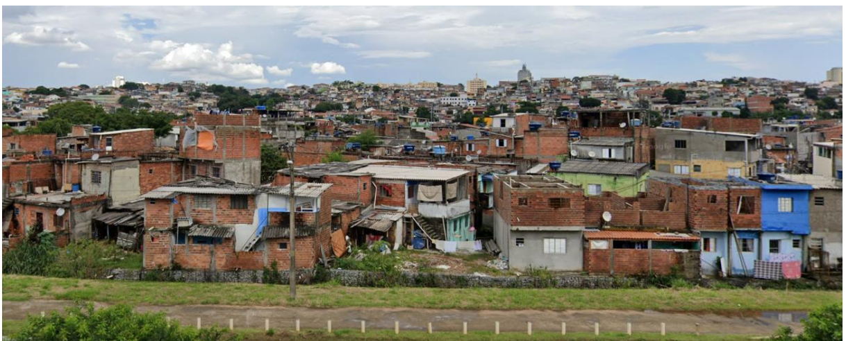
Figure 24: Example 3 of very high risk to flood events - Jardim Piratininga in São Paulo. Source: Google Maps, 2022.
