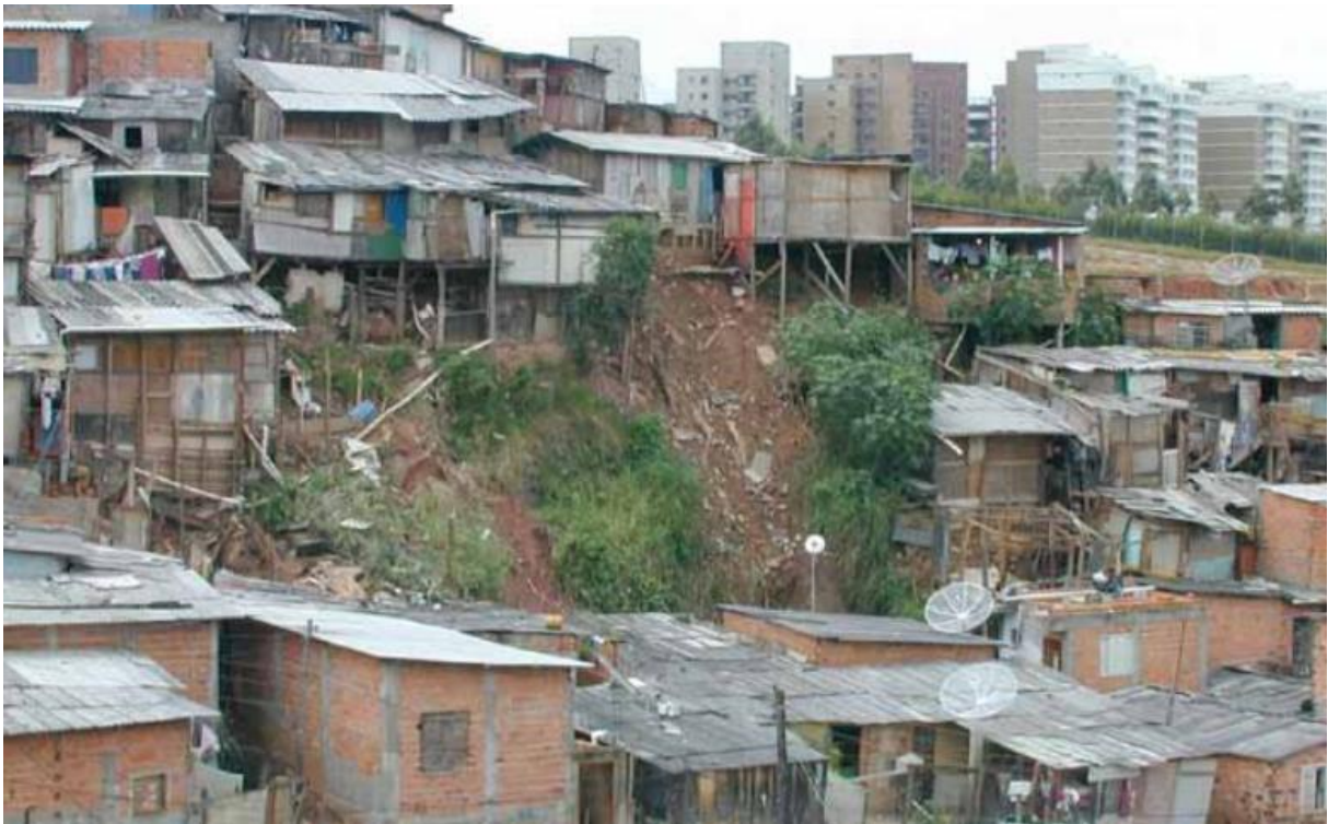
Figure 9: Precarious settlement classified as landslide risk area. Photo: IPT, 2010. Source: Nobre et al., 2010.
