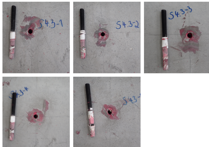
FIGURE C.99: S4.3-C - Failure of the anchors
