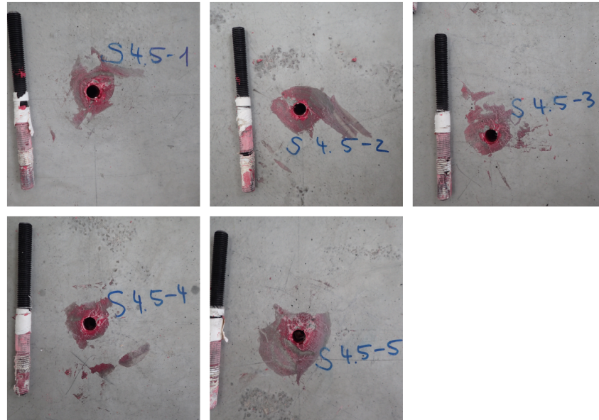
FIGURE C.107: S4.5-C - Failure of the anchors
