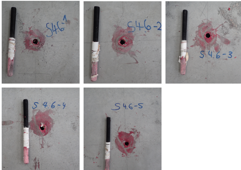
FIGURE C.109: S4.6-C - Failure of the anchors
