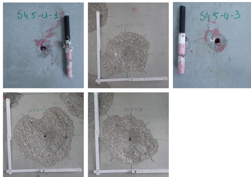
FIGURE C.108: S4.5-U - Failure of the anchors
