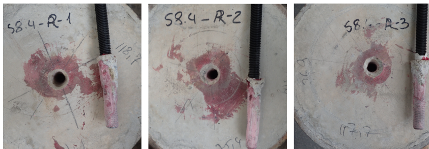
FIGURE C.127: S8.4-R - Failure of the anchors
