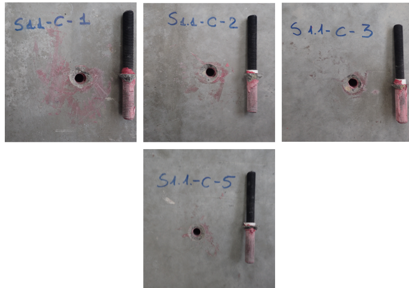
FIGURE C.66: S1.1-C - Failure of the anchors
