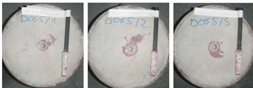
FIGURE B.112: D051 - Failure of the anchors
