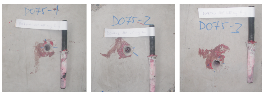
FIGURE B.119: D075 - Failure of the anchors
