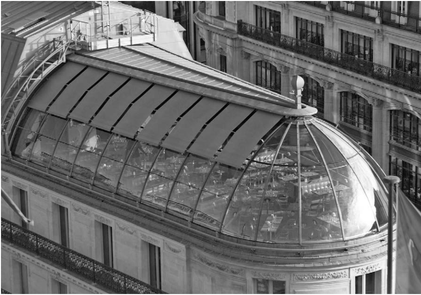
Figure 6.3: Kong Bar-Restaurant in Paris with external shading system. 18 blinds protect this glass roofing and absorb 97% of the sun's heat. Interestingly, however, this system has geometrical limitations and cannot easily be applied to the double-curved areas of the facade.
