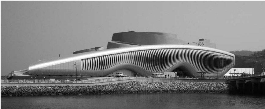
Figure 6.30: Ocean One pavilion at the Expo 2012 in Yeosu features a kinetic facade with 108 bendable lamellas that allow for controlled light exposure of the facade.
