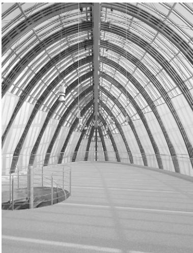
Figure 6.4: Shading system inside the double-curved facade of the Peek & Cloppenburg building.
