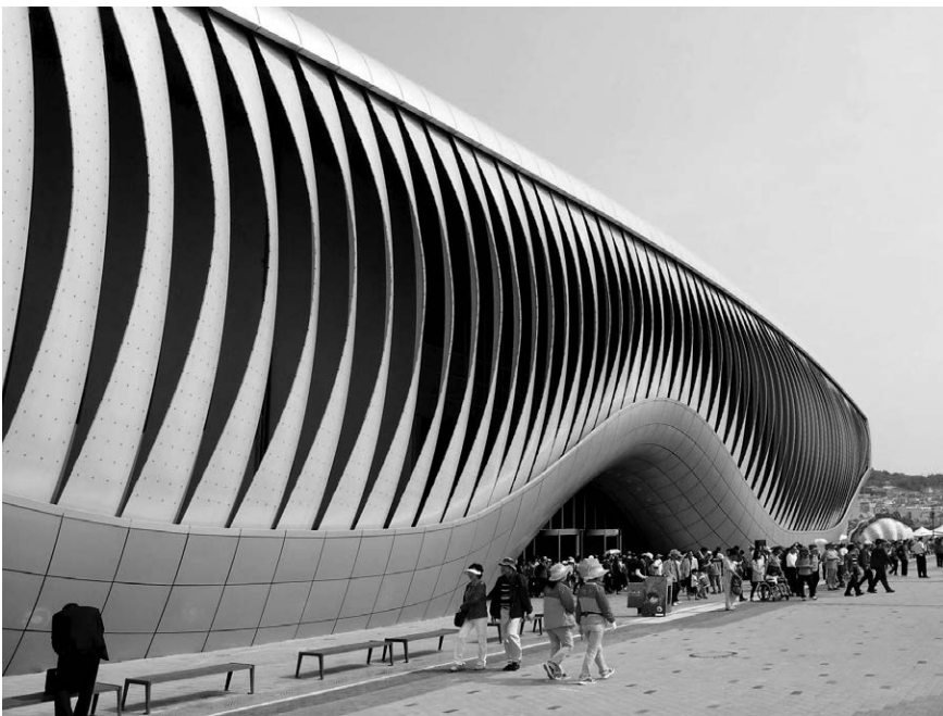
Figure 6.31-6.32: The up to 14 m high lamellas can be opened and closed individually and thus enable an impressive transformation of the building envelope.
