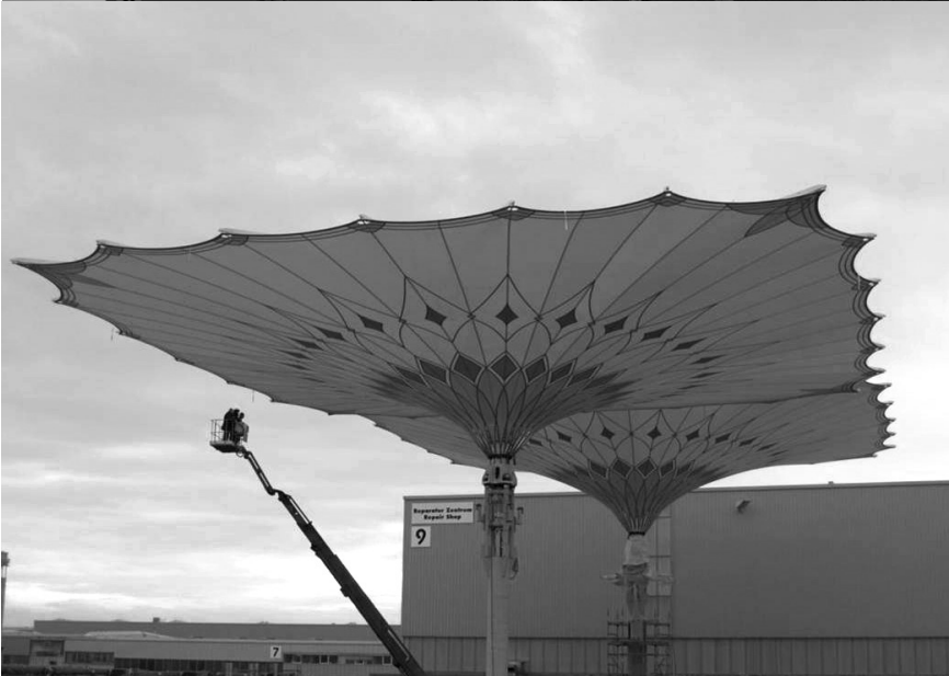
Figure 2.12: Construction of large convertible umbrellas. The retractable arms in this umbrella structure feature a parallelogram mechanism with a four-bar linkage.
