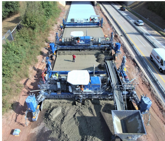
Figure 3. Two-layer concrete paving and spraying.
